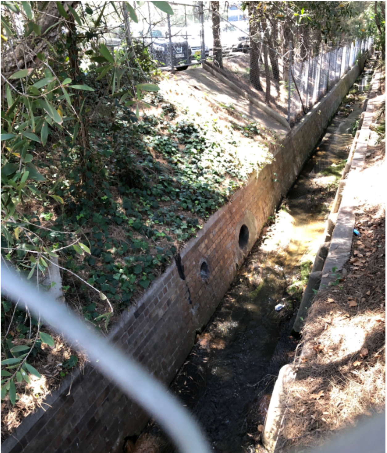
Figure 2 Existing Sydney Water Channel
