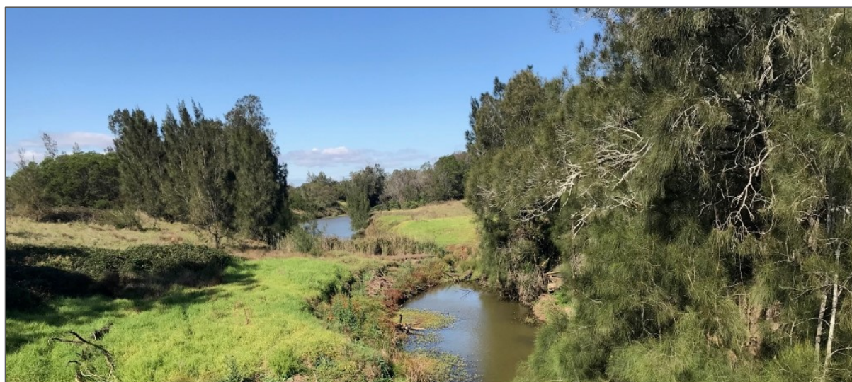
Figure 4: South Creek at the subject land. Historical weir/crossing can be seen mid-image with upstream weir pool.
