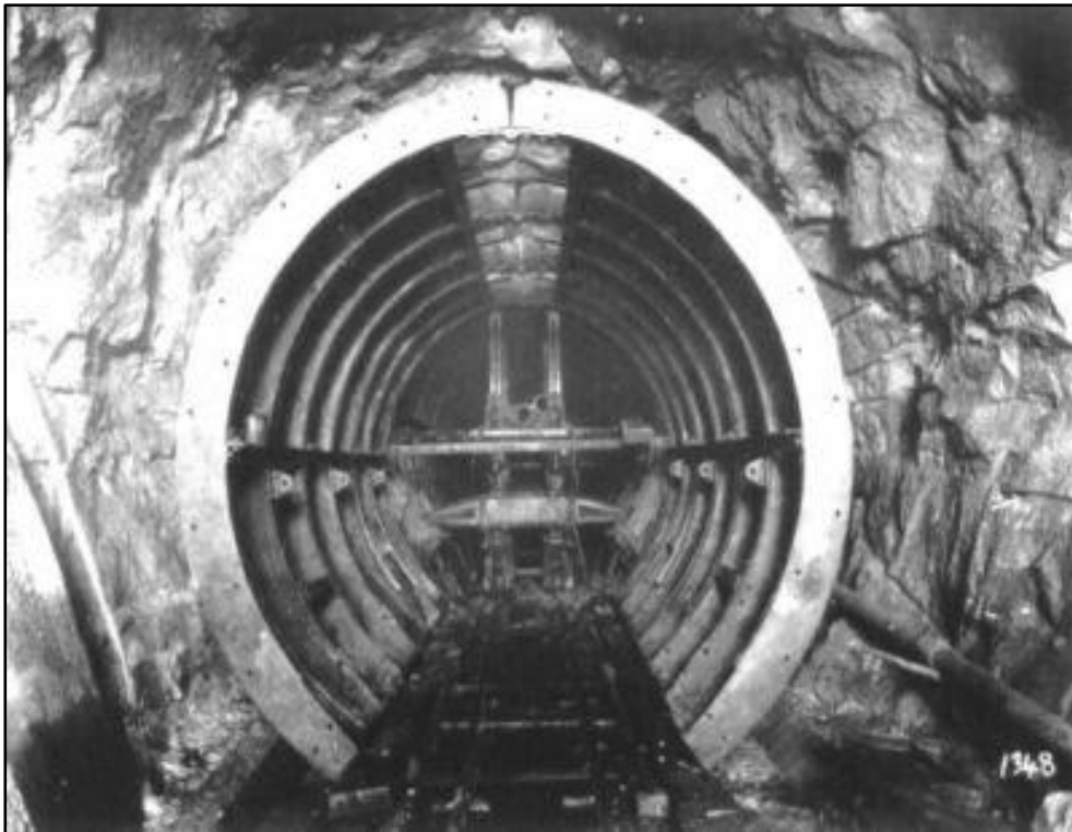
Figure 43: Pressure Tunnel formwork 162
