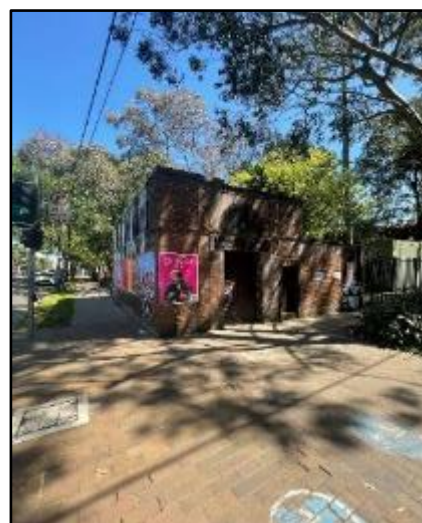
Figure 86: SU2 – Electricity Substation (LEP no. I2086) along McEvoy Street, view northwest
