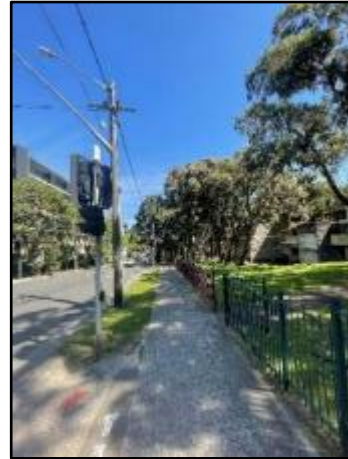
Figure 88: SU4 – Concrete footpaths and front yards of social housing, view west along McEvoy Street showing declining slope
