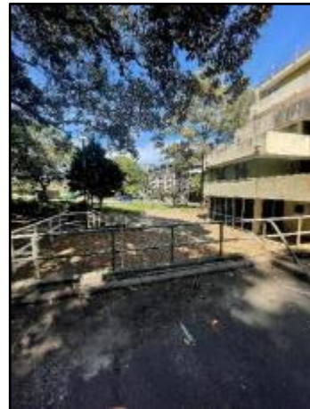
Figure 90: SU4 – social housing cut into natural slope, view south
