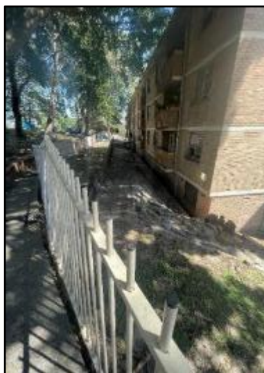
Figure 96: SU5 – social housing cut into natural slope, view south
