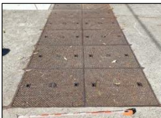
Figure 74: SU1 – subsurface services along concrete footpath
