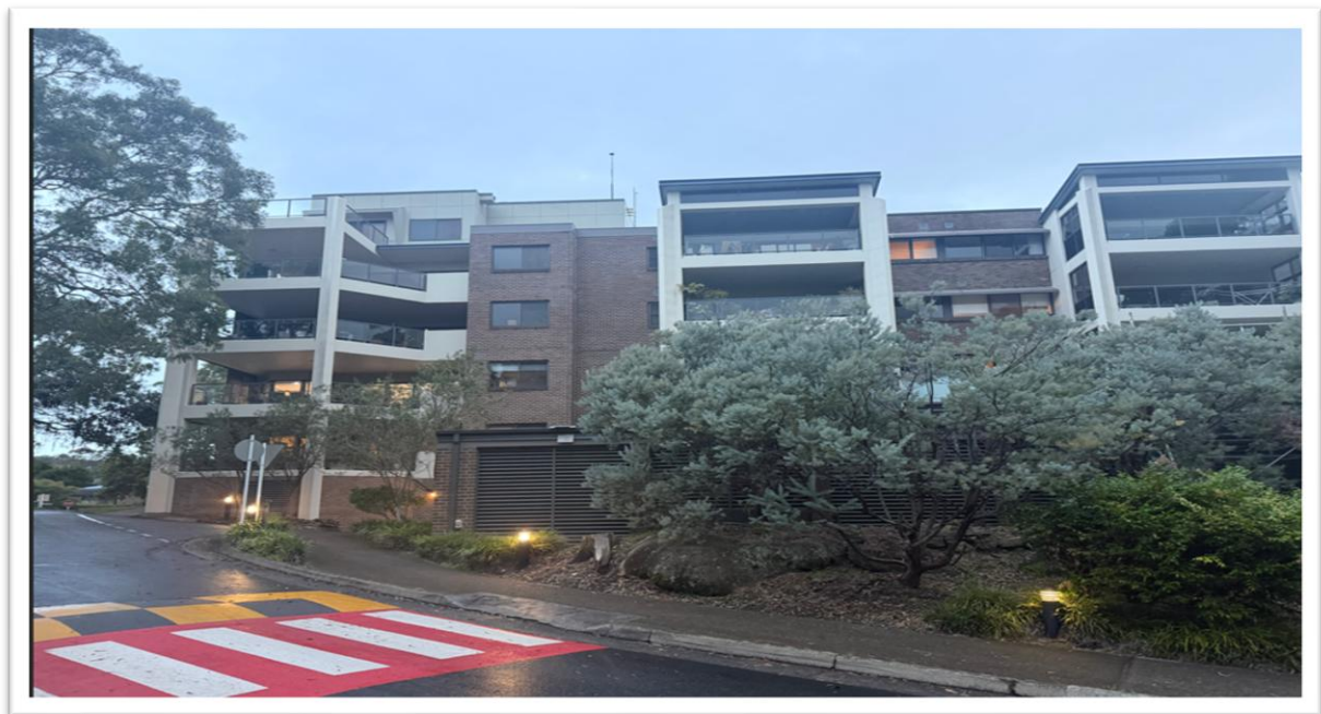
Figure 4 - Existing 6 story building on site in close proximity to proposed staged 1 and below existing tree canopy.
