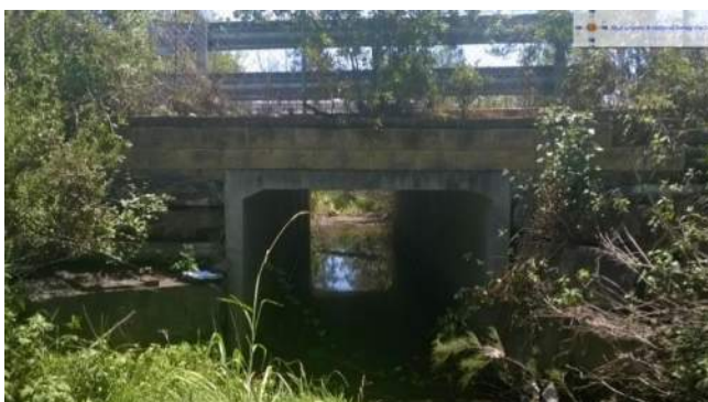
Culvert at site access road (upstream side)
