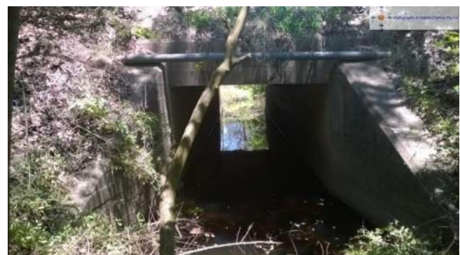
Culvert at rail lines (upstream side)
