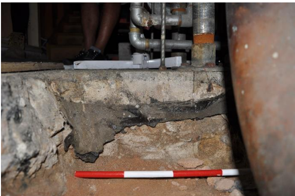
Figure 4.5 Concrete slab constructed onto the sandstone bedrock. (Source: GML, 2019)
