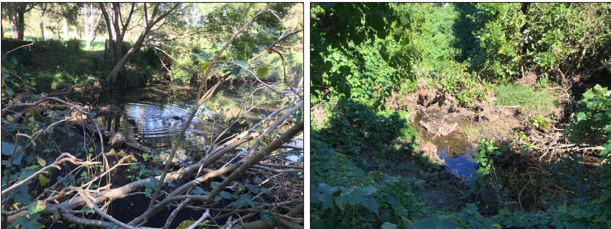
Figure 3-15 Burnt Bridge Creek spilling weir with deep pool (left). Constricted middle reach downstream (north of Balgowlah Road), heavily constricted by exotic weeds and trees (right) (Photo date: 26/05/2021).
