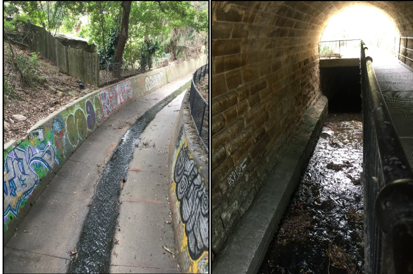
Figure 3-3 Flat Rock Creek concrete lined areas (left) and along the underground channel (right) (Photo date: 27/05/2021).
