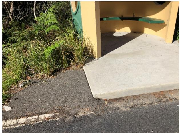
**Figure 2-6 Interior of bus shelter and newly concreted ramp and interior**
