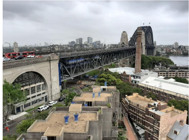
Figure 18 -The Sydney Harbour Bridge from level 11 of the Sirius building .
