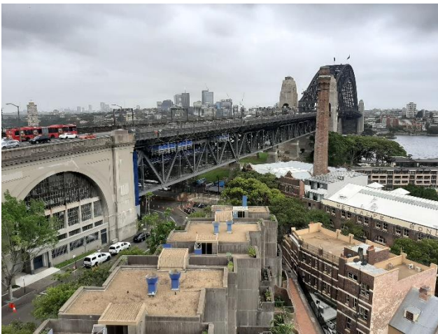
Figure 8 - View north west of the Sirius building with Bradfield highway between Sirius and Millers Point
