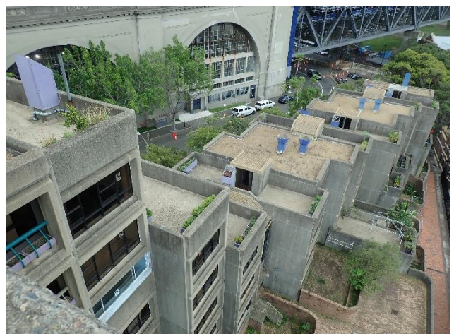
Figure 16 – stepping down of the roof of Sirius to the north.
