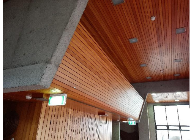
Figure 12 – Panelling on roof of foyer inside the building.
