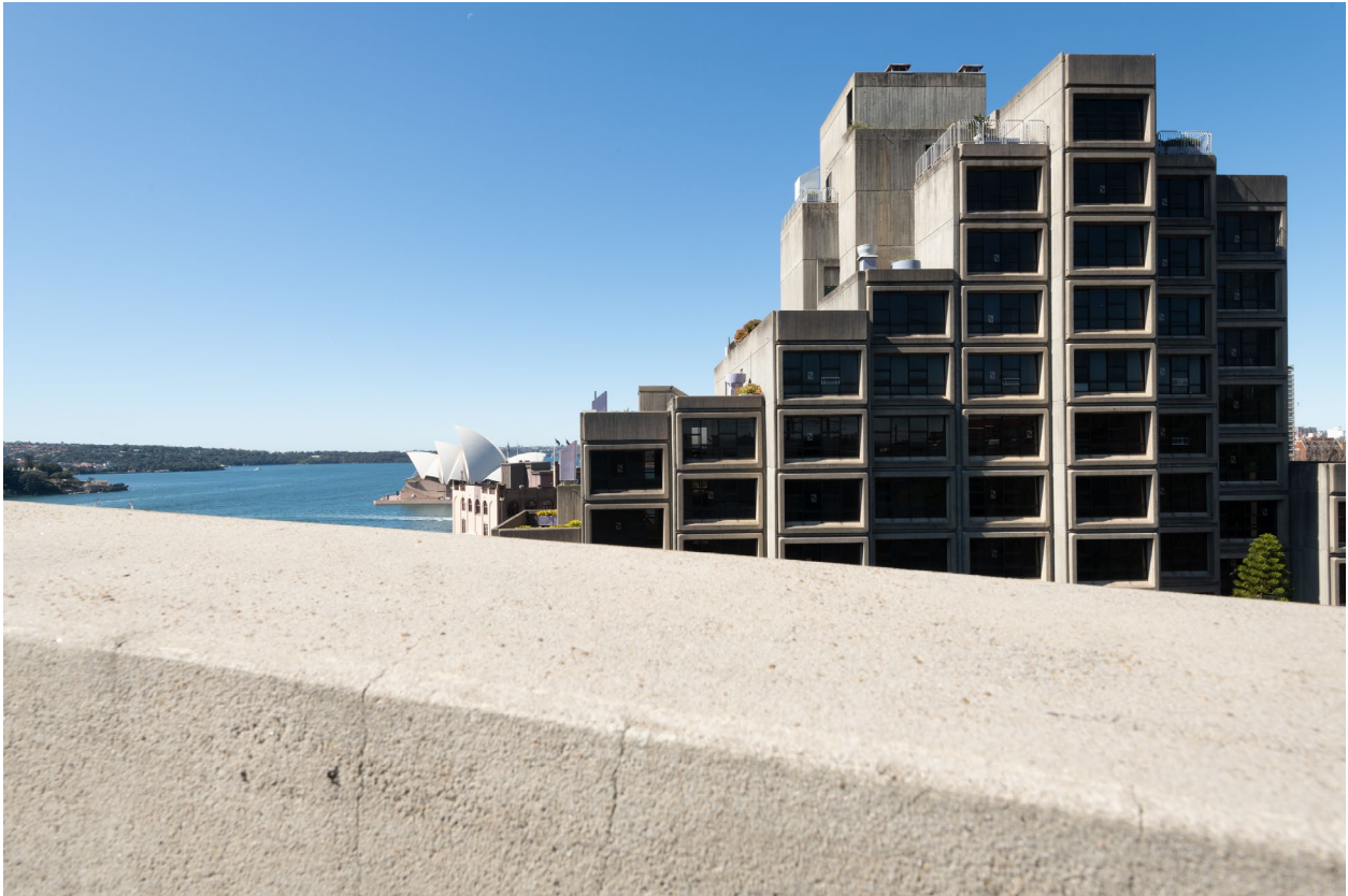
Wider version of View I04 (existing condition) captured using a 20mm lens (Modata).
