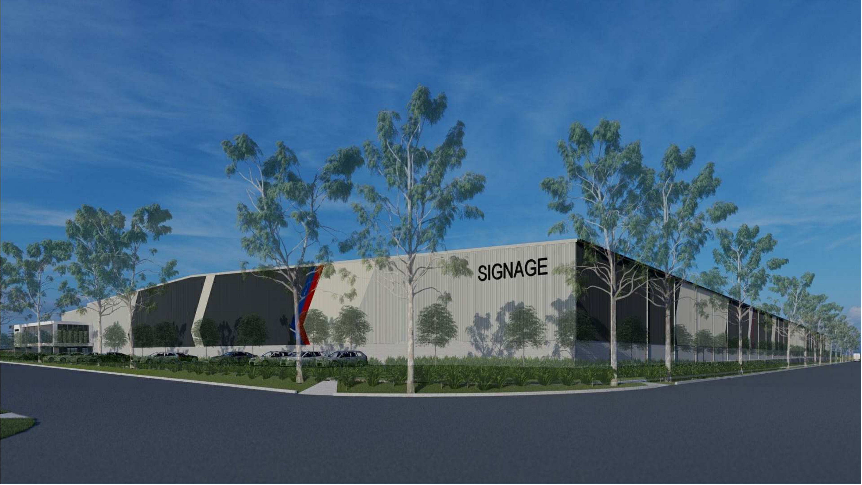
BUILDING WH5 SOUTH - EAST VIEW
