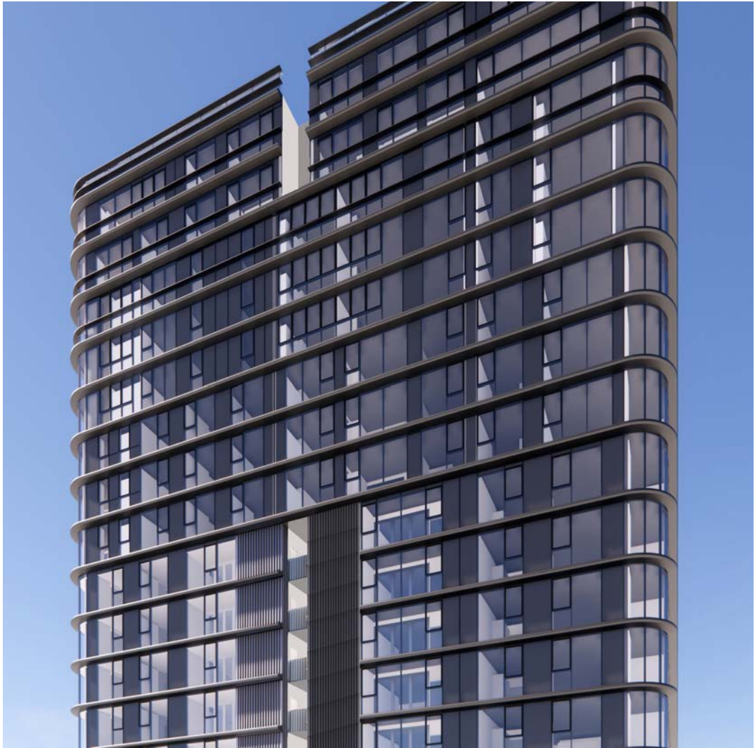
View of Cottonwood Tower Southern Facade
