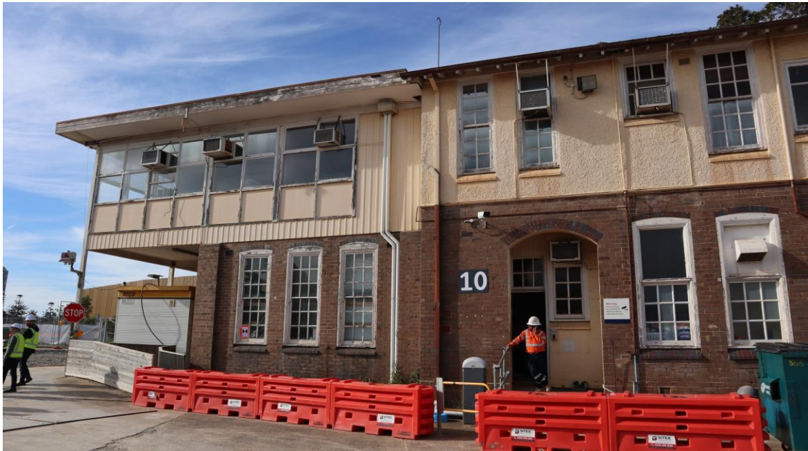
Figure 30: West Elevation Mowbray House, viewed from within the site.
