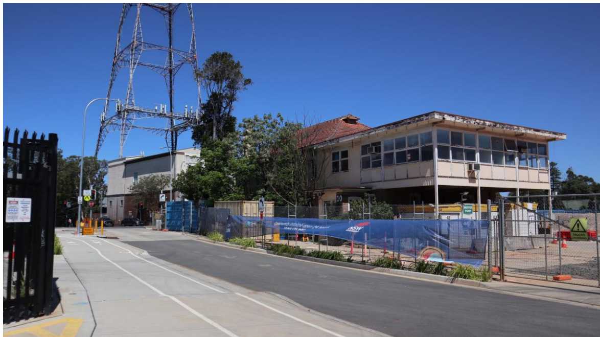
Figure 29: North East Elevation Mowbray House, viewed from Frank Channon Walk
