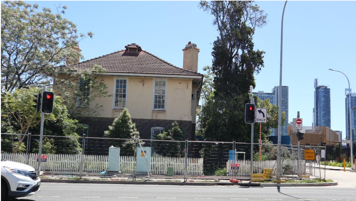
Figure 81. The view north towards the subject site from Hampden Road and Mowbray Road.
