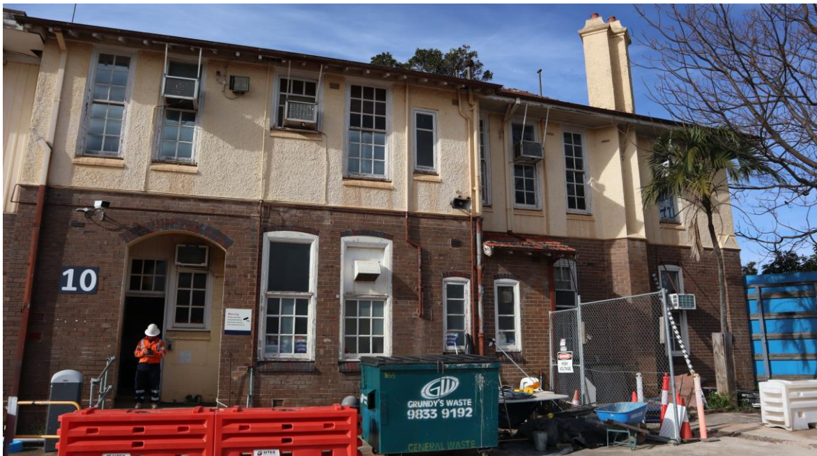
Figure 31: West Elevation Mowbray House, viewed from within the site.
