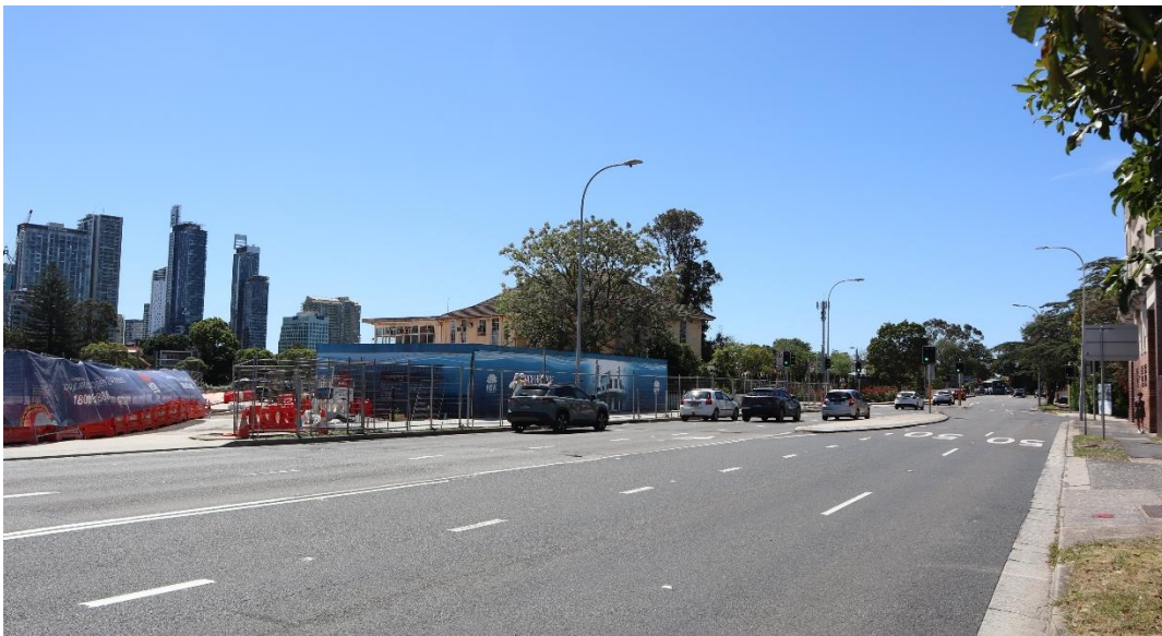
Figure 21: Mowbray Road, looking East. Subject site on the left.
