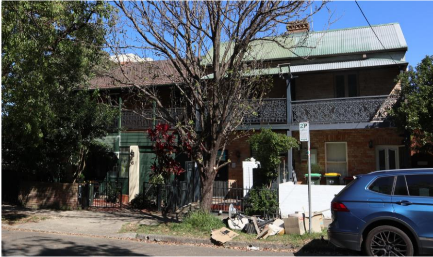
Figure 40: The Terrace House, viewed from Moriarty Road.
