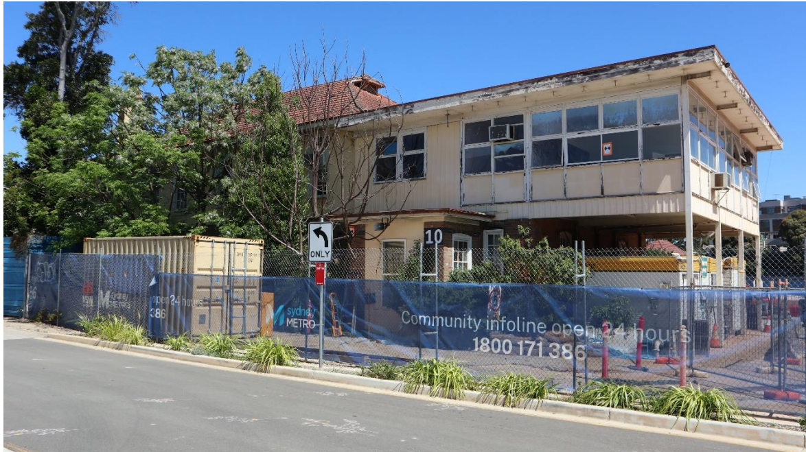
Figure 28: East Elevation Mowbray House, viewed from Frank Channon Walk
