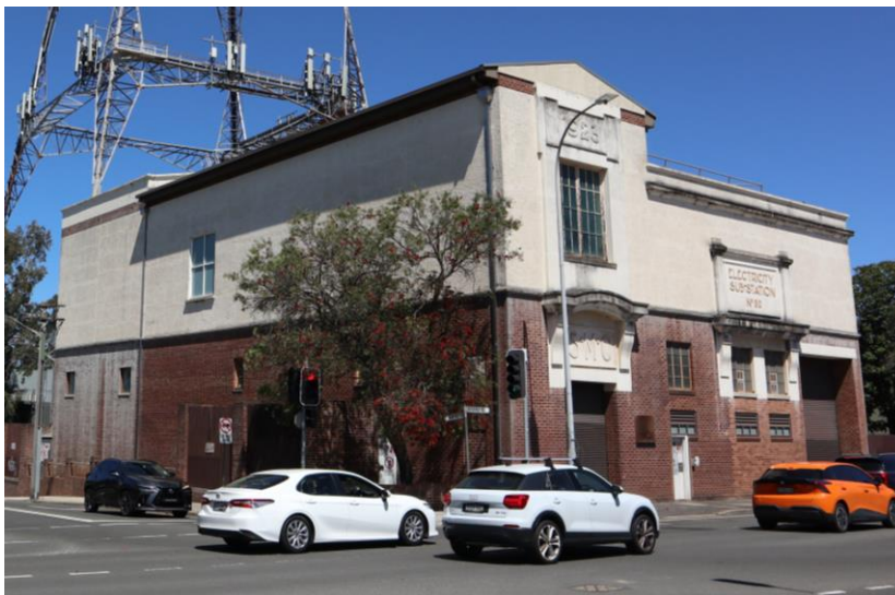
Figure 39: The Chatswood Zone Substation No.80, viewed from Mowbray Road
