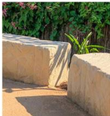
FN01 - SALVAGED SANDSTONE BLOCK SEATING
