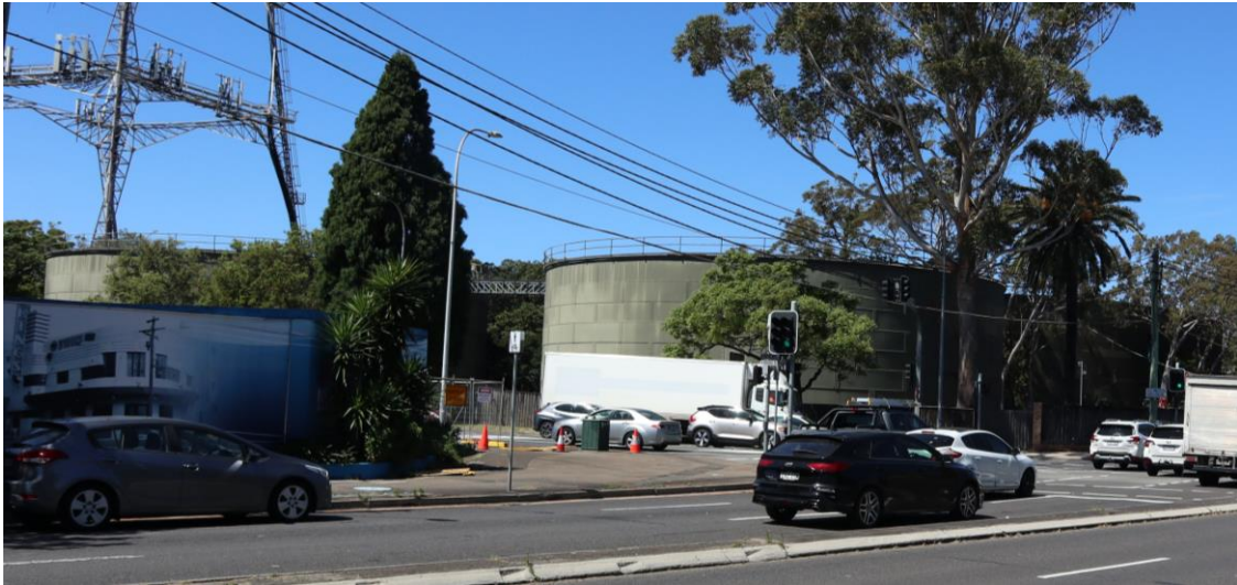
Figure 35: Chatswood Reservoirs, viewed from Pacific Highway
