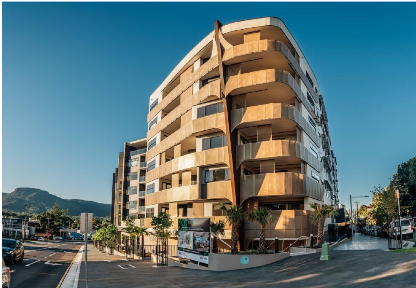
Figure 22 Mt Keira seen in the background of a view from the adjoining public space
