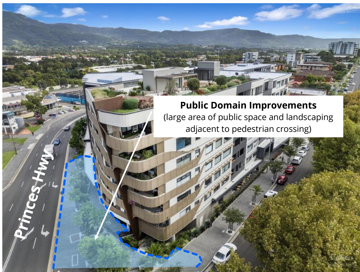
Figure 23 Aerial photograph of the new public space at the north-east corner of the Princes Highway, Smith Street and Keira Street
