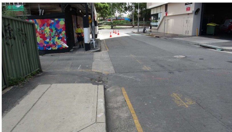
Photo taken in 2021 showing the barrier kerb and a dish gutter at the entrance to William Lane. During the minor storm event, floodwater will be flowing toward Gibbons St at the background, without entering William Lane. The 2020 Lidar terrain and contours did not display drainage feature of this small dish gutter.
