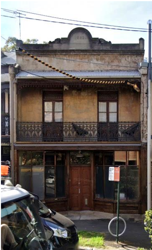
Figure 17. Google Street View image of 189 Pitt Street, Redfern. No interior images could be located.
