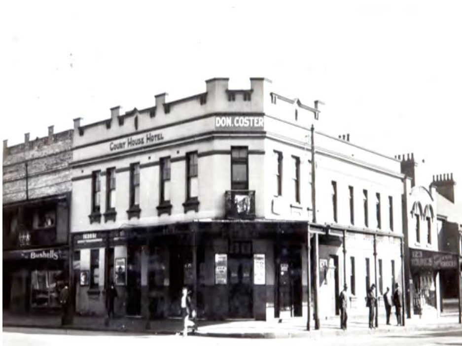
Figure 8: 1930s image of the former Court House Hotel. 64
