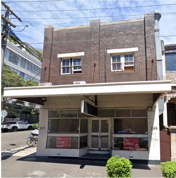
Figure 61. Google Street View image of 265 Cleveland Street, Redfern.
