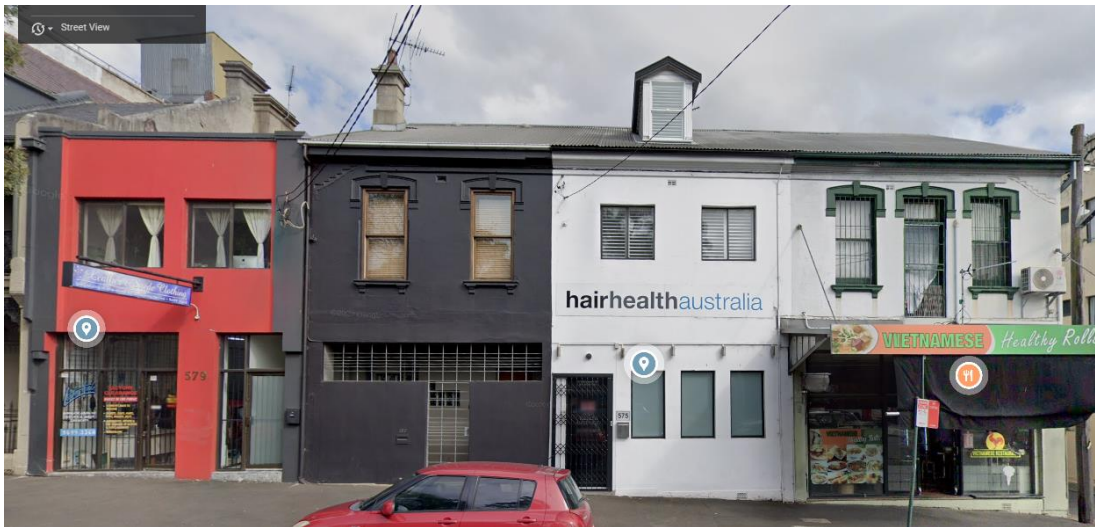
Figure 59. Google Street View image of 573–579 Elizabeth St, Redfern.
