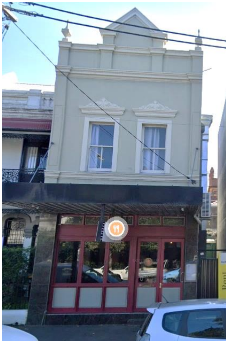
Figure 34. Google Street View image of 96 Pitt Street, Redfern.
