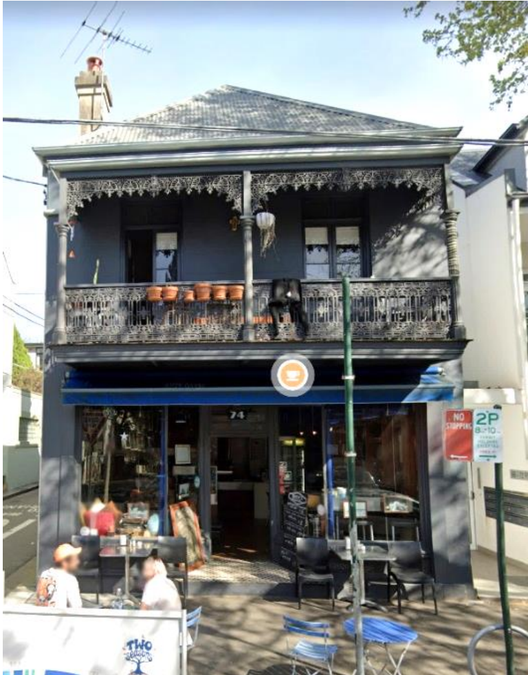
Figure 31. Google Street View image of 74 Pitt Street, Redfern.
