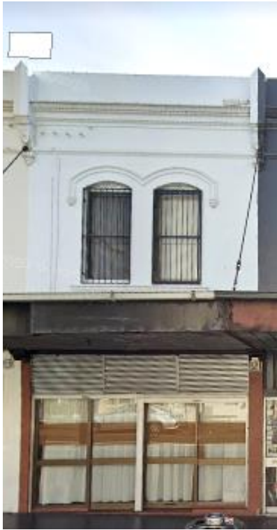
Figure 50. Google Street View image of 90 Redfern Street, Redfern. No interior images could be located.
