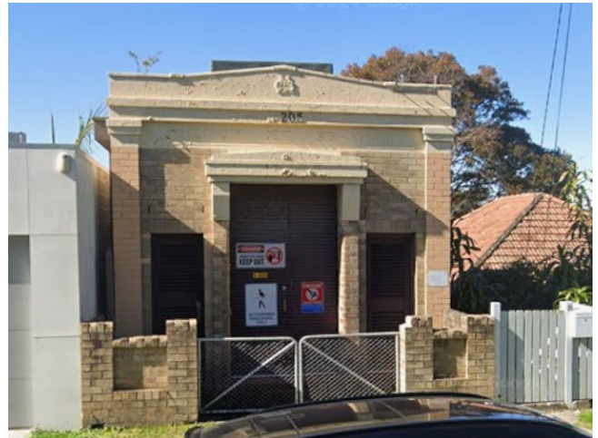
Figure 15 Electrical Substation 205, Redan Street.
