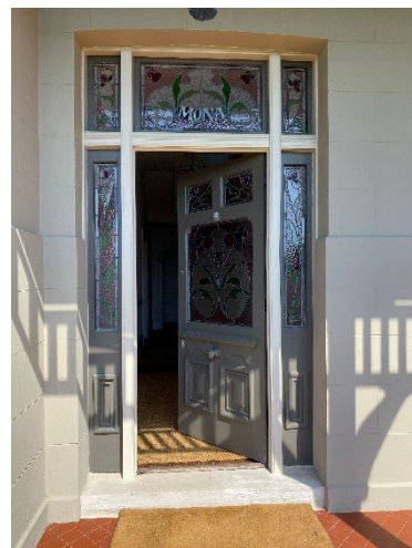
Figure 34 Front door at the primary entrance from Redan Street.
