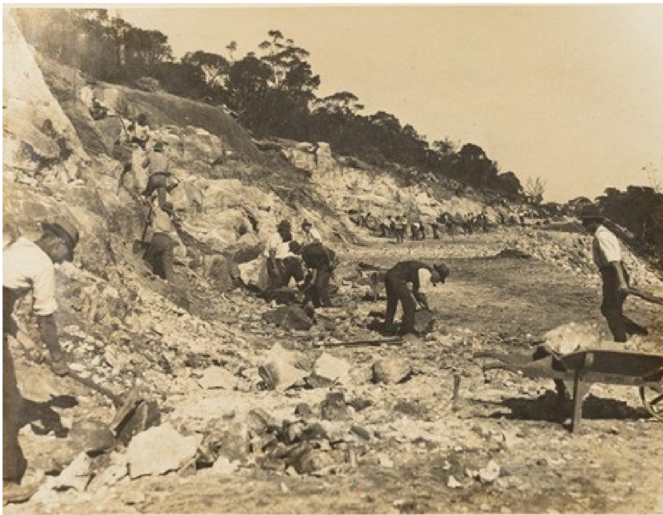
Figure 81 1922 example of the road under construction in Mosman. Note the steep terrain.
