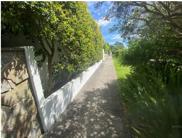
Figure 43 Concrete fence with built in garden bed of 48 Redan Street.
