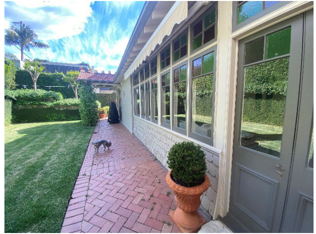
Figure 36 External view of the southern extension.
