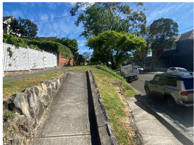
Figure 9 Retaining wall, with the Divided Road to the right.
