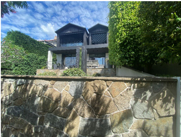
Figure 41 Primary façade of 46 Redan Street.
