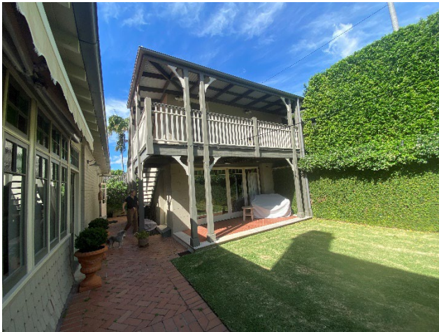
Figure 37 Ancillary structure located to the rear of the house.
