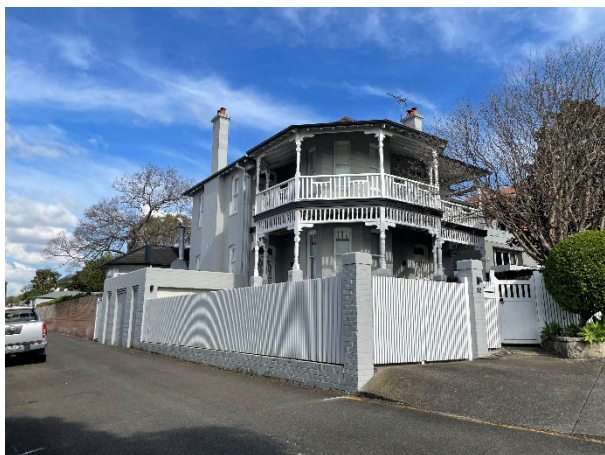
Figure 114 52 Almora Street, on the corner with Redan Lane, showing its primary address towards Almora Street.
