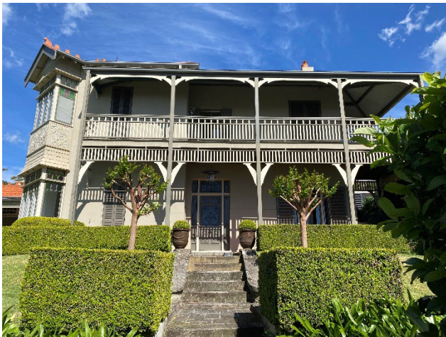
Figure 31 Primary façade of 44 Redan Street.
