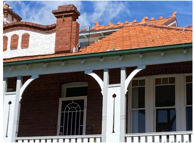
Figure 11 Detail of the roof of 38 Redan Street.
