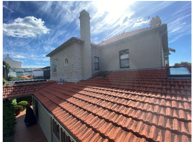
Figure 38 View across the roof, showing orange terracotta tiles.
