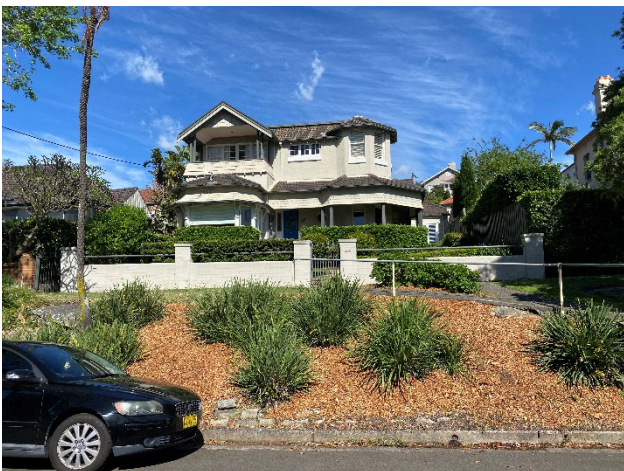
Figure 25 Primary façade of 42 Redan Street. Note the retaining wall that separates the house from the street.
