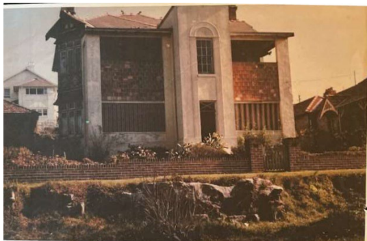
Figure 71 44 Redan Street in 1960s showing eastern façade at the time of buildings use for two flats.
