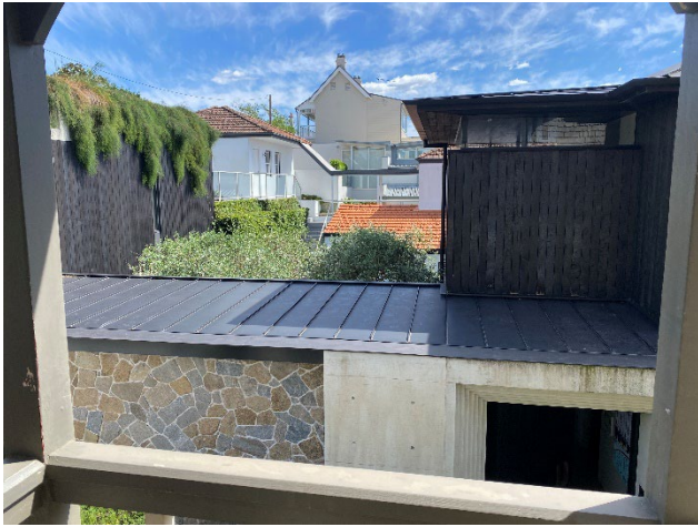
Figure 39 Covered extension of 46 Redan Street, as seen from 44 Redan Street.
