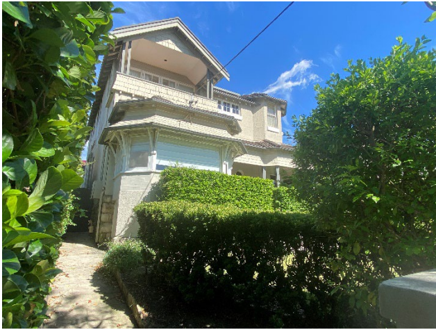
Figure 27 Southern corner of the primary elevation.
