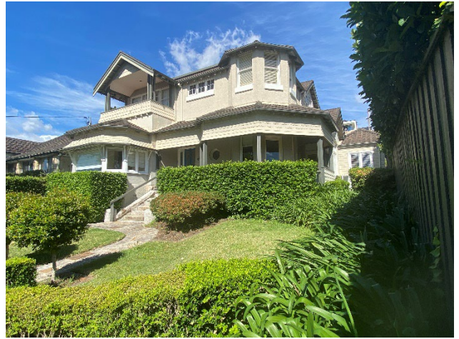
Figure 28 42 Redan Street, addition to the house seen in the background (right).
