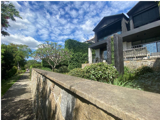
Figure 42 Primary façade showing stonework detail of the podium.
