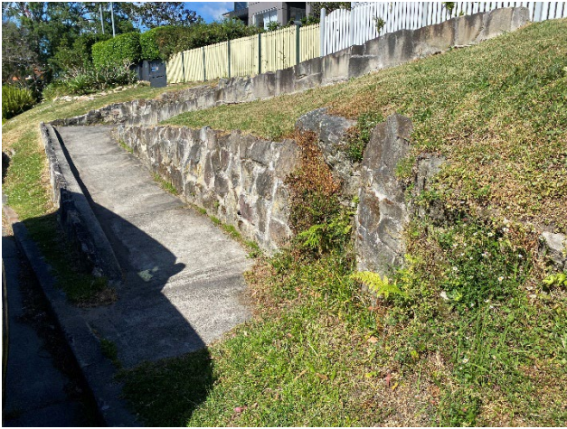
Figure 23 Concrete path cut into the retaining wall in front of 40 Redan Street.
