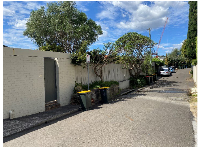
Figure 30 Rear access to 42 Redan Street from Redan Lane.
