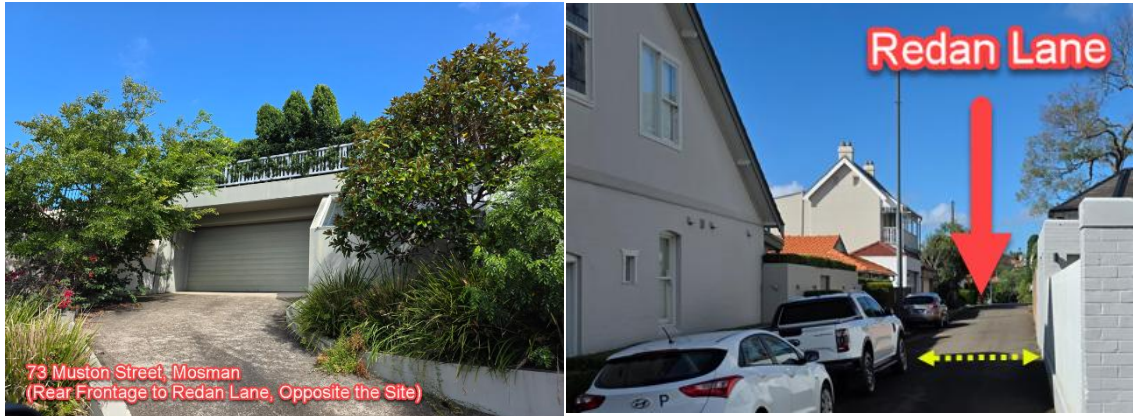
Figure 2 73 Muston Street (Left) and Narrow Redan Lane (Looking South) with No Pedestrian Footpath (Right)
