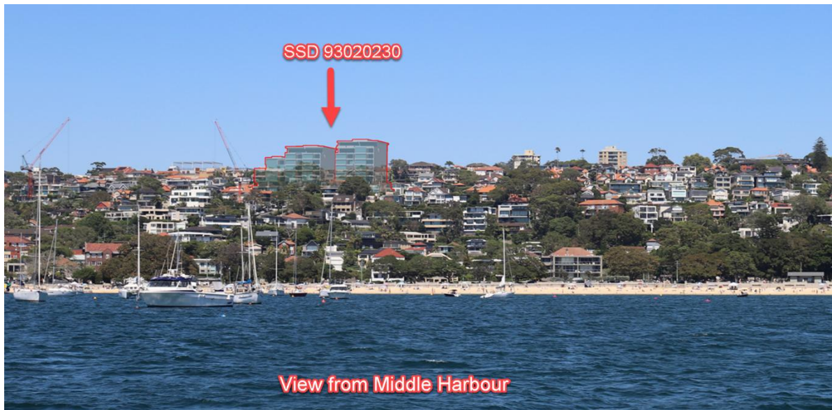
Figure 18 Significant Visual Impact When Viewed from Middle Harbour (Pam Walls 50mm focal length 08/01/2026 10:48)
