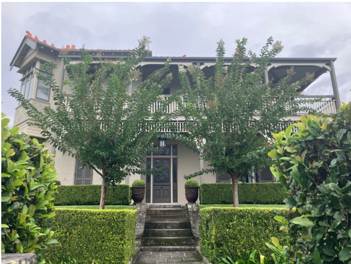
Figure 10: Existing building located at 44 Redan Street proposed for demolition.
