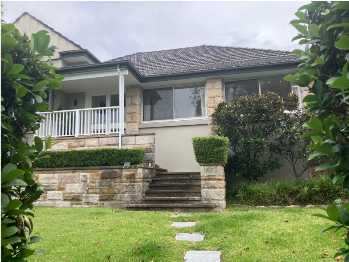
Figure 8: Existing building located at 40 Redan Street proposed for demolition.
