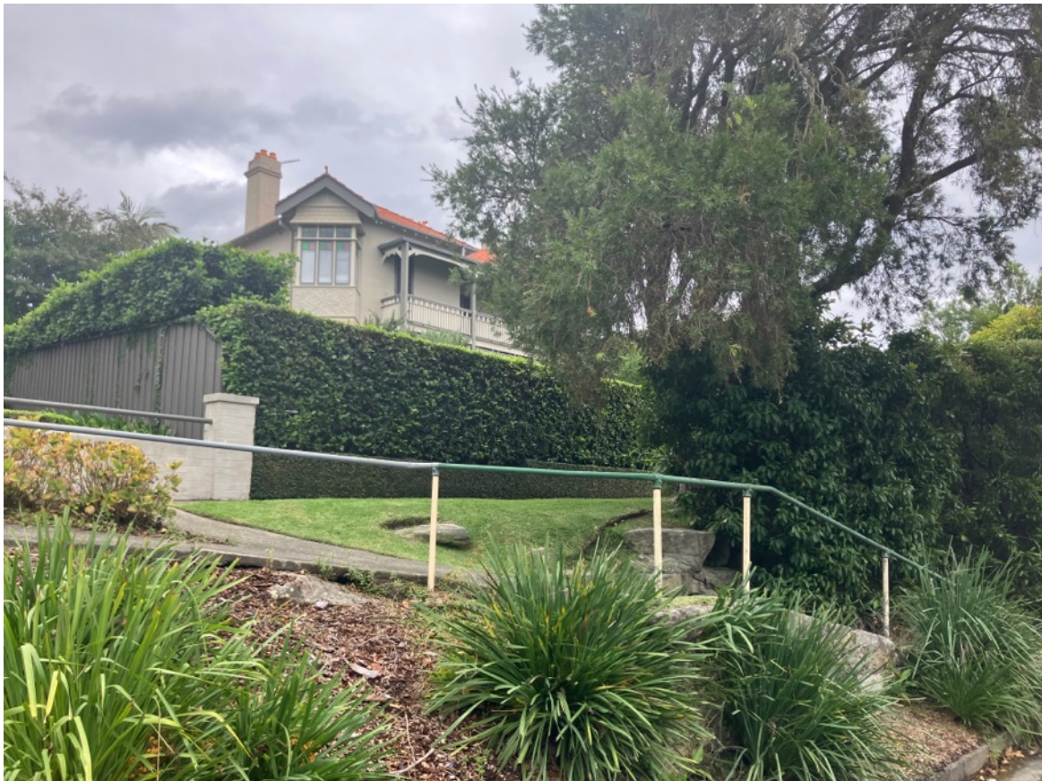
Figure 6: Heritage listed Redan Street embankment and landscape features.
