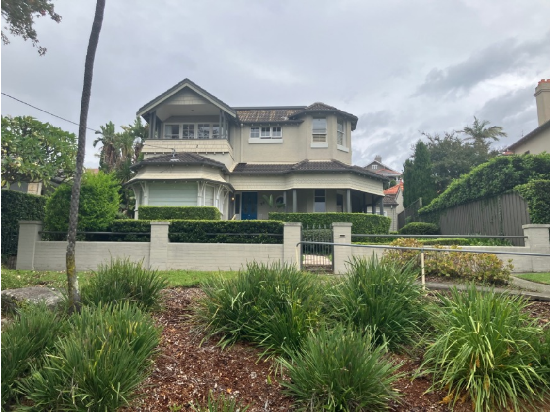
Figure 9: Existing building located at 42 Redan Street proposed for demolition.
