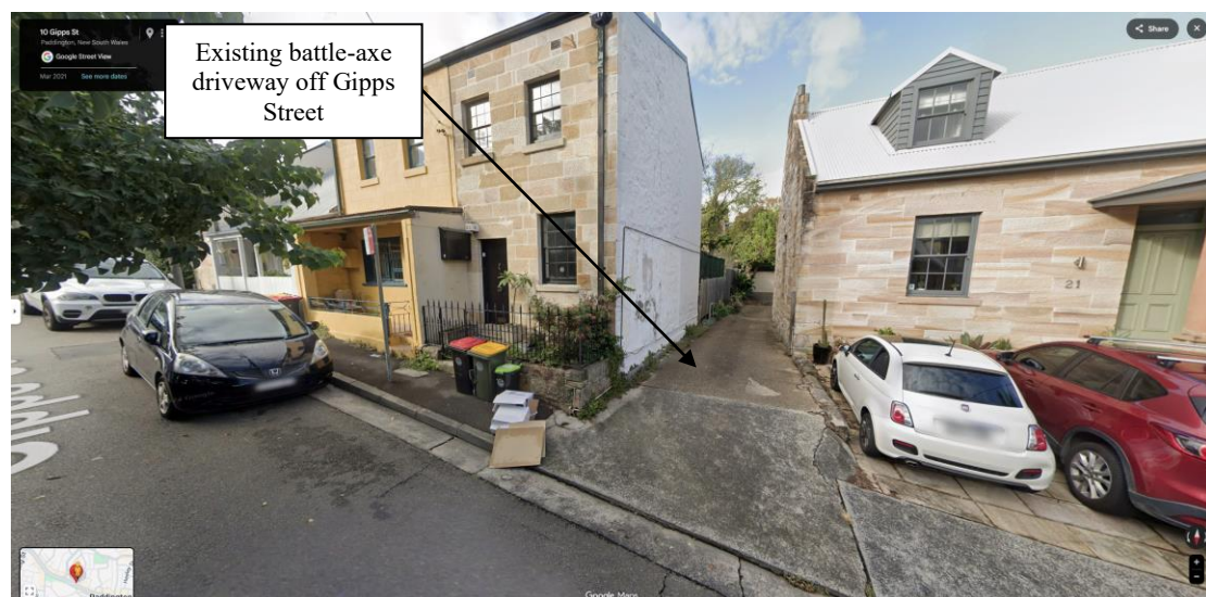
Site viewed along the Gipps Street site fronting, outside the battle-axe driveway
