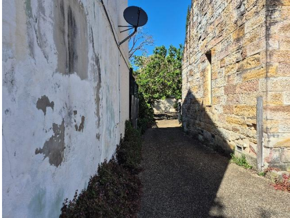
Figure 29. Lane Access from Gipps St Looking south.
