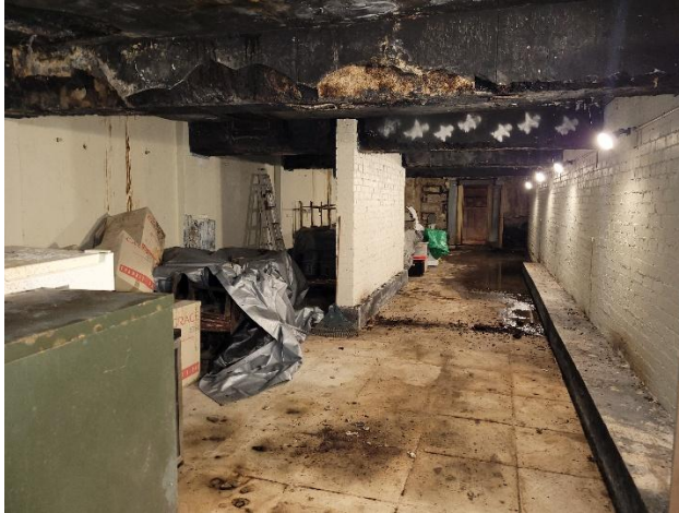
Figure 36. The largest room within the basement with small internal dividing wall. View to the north.
