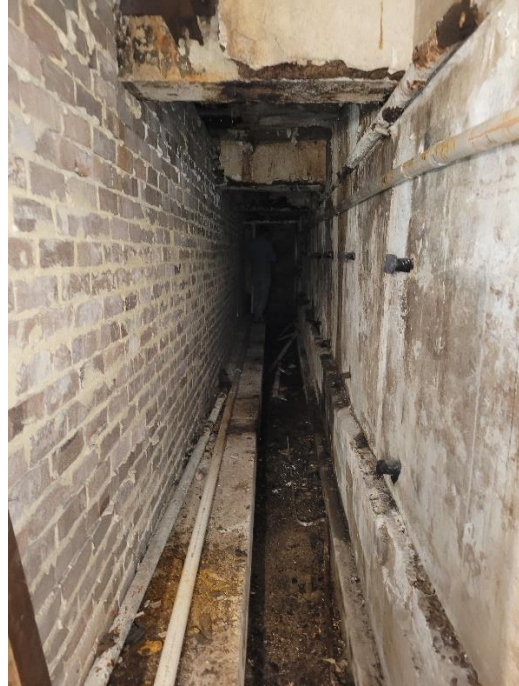
Figure 37. View to the north showing drainage channel running along corridor.
