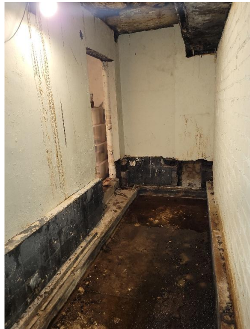
Figure 35. Corridor dividing the basement stairs from the largest room. View to the west.
