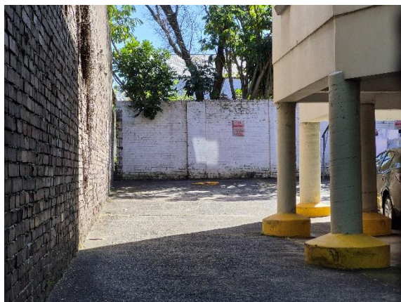
Figure 25. Carpark. View to the north.
