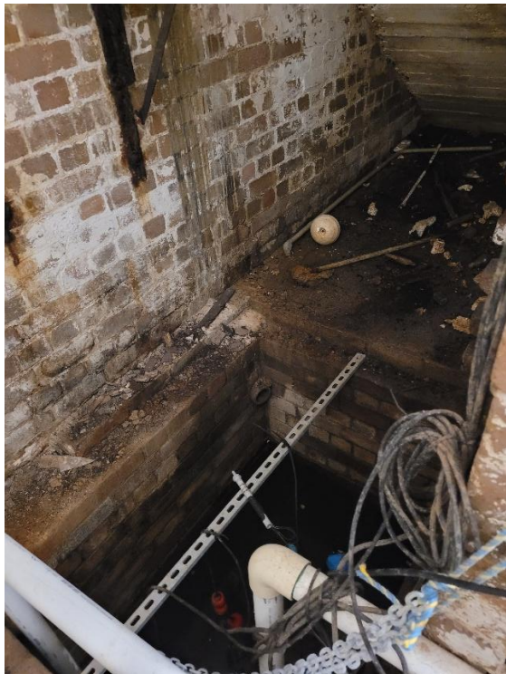
Figure 38. Sump below the stairs. View to the southwest.
