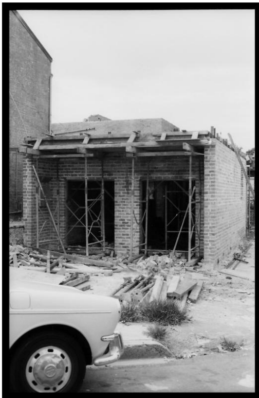
Figure 20. Construction of 13 Gipps Street in 1982 (National Trust).
