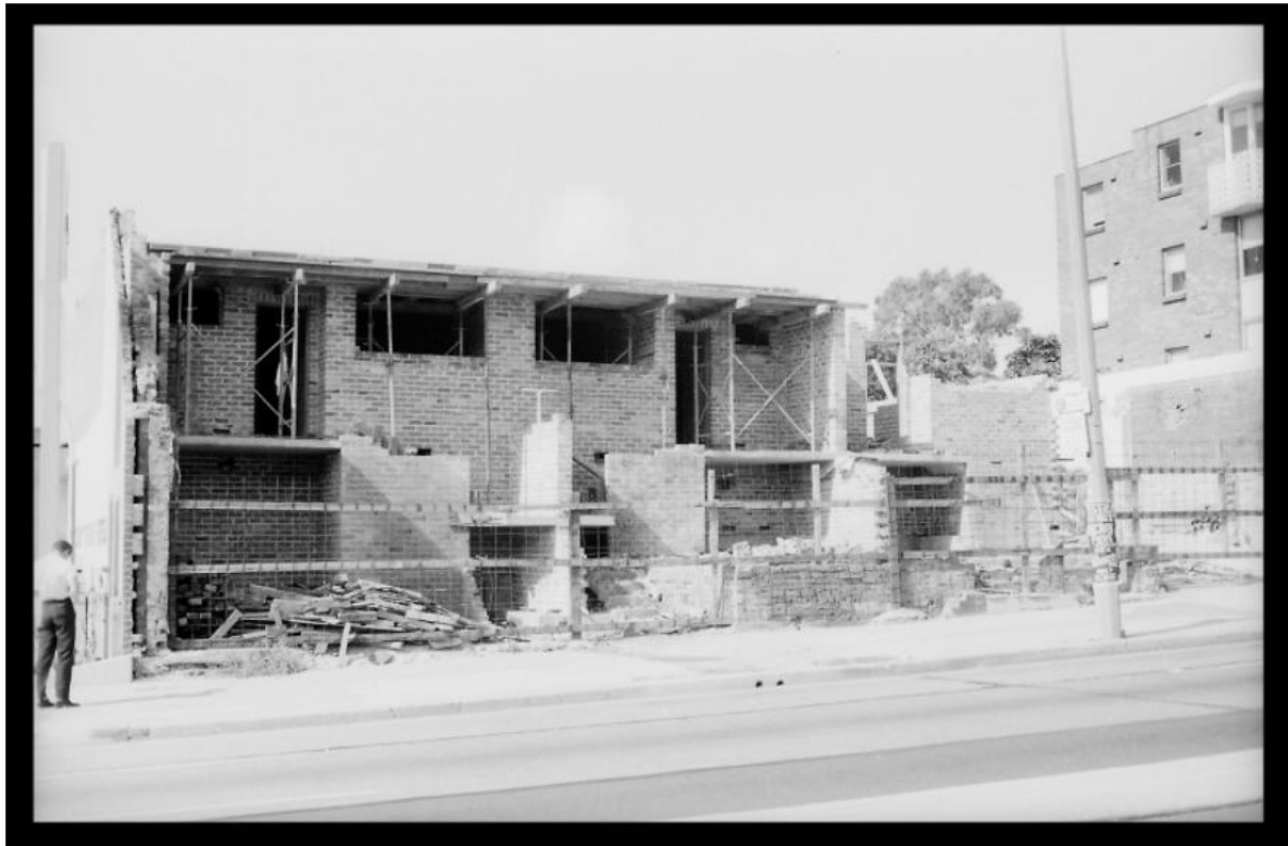
Figure 20. Construction of 142-148 Oxford Street in 1982 (National Trust).
