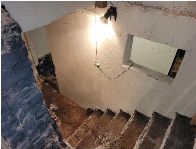
Figure 34. Stairs leading down to the basement level, looking northwest.
