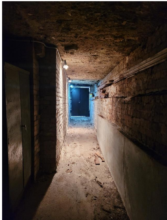
Figure 39. Corridor leading to the courtyard parking area. View to the west.
