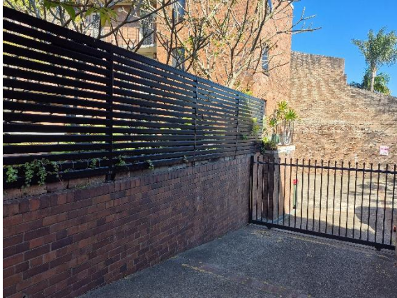
Figure 27. Bottom of the ramp with elevated courtyard at the left.
