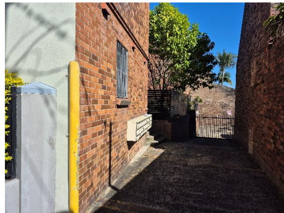
Figure 22. Entrance on Shadforth St.
