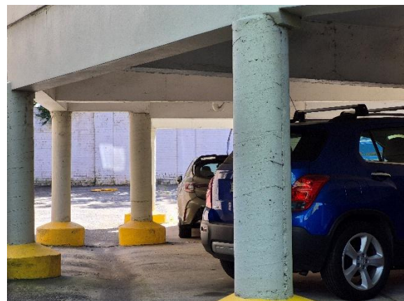
Figure 26. Detail of piles. View to the northeast.
