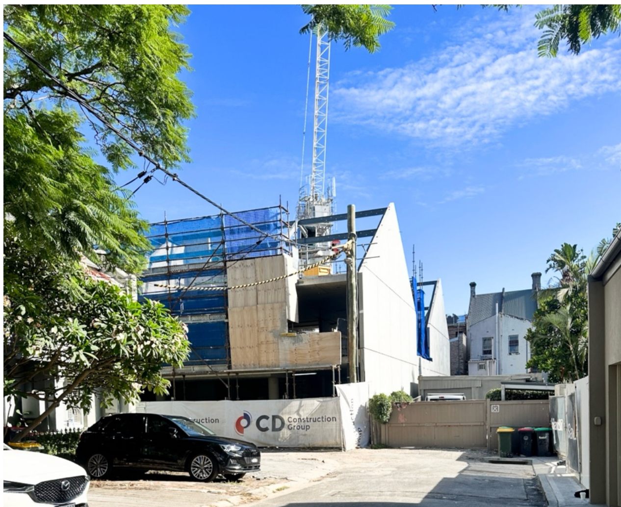
432–440 Oxford from rear. Currently under construction
