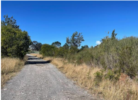
Figure 9: Internal access road, view east
