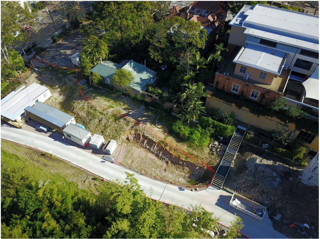
Figure 2 - 50 McLaren Street and southern end of 52 McLaren Street : (Source: Wenona)
