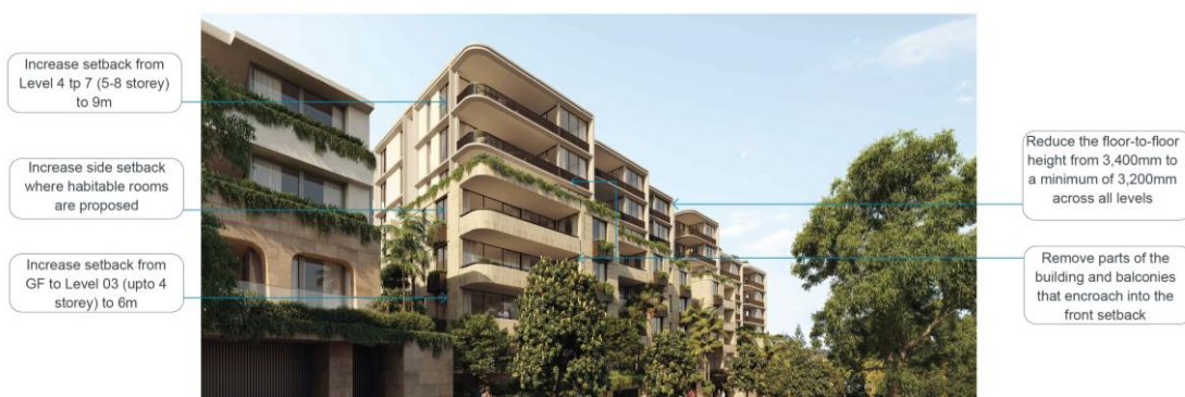
Figure 4 – Summary of key recommendations for western boundary shown over Photomontage 02 by MHNDU
