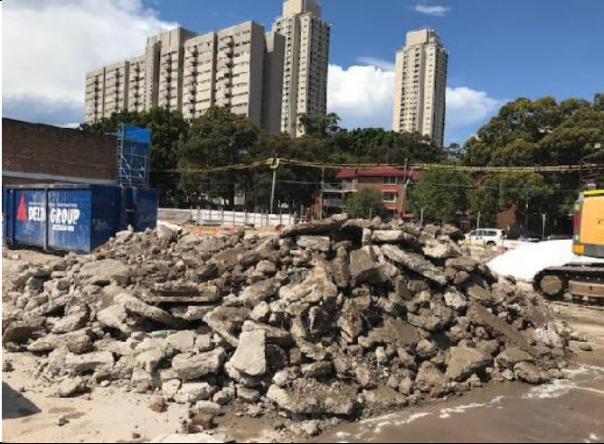
Photo 1: Central section of site, adjacent to site sheds following Sparrow pick of asbestos containing debris within bulk concrete stockpile
