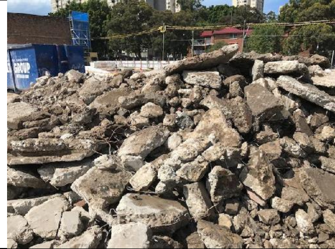
Photo 2: Central section of site, adjacent to site sheds following Sparrow pick of asbestos containing debris within bulk concrete stockpile
