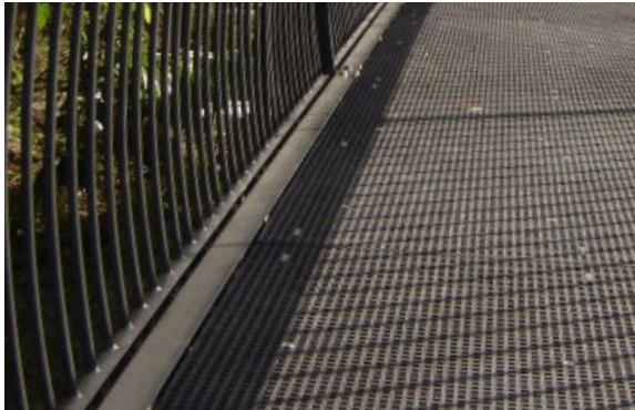
GRP Decking to pedestrian ramp
