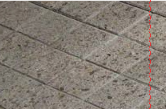
Interlocking concrete unit paver (vehicular grade)
