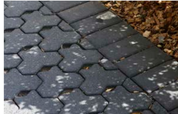
Eco Tri Hex Permeable Paver
