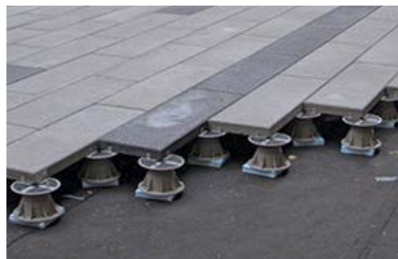
Concrete pavers on pedestals
