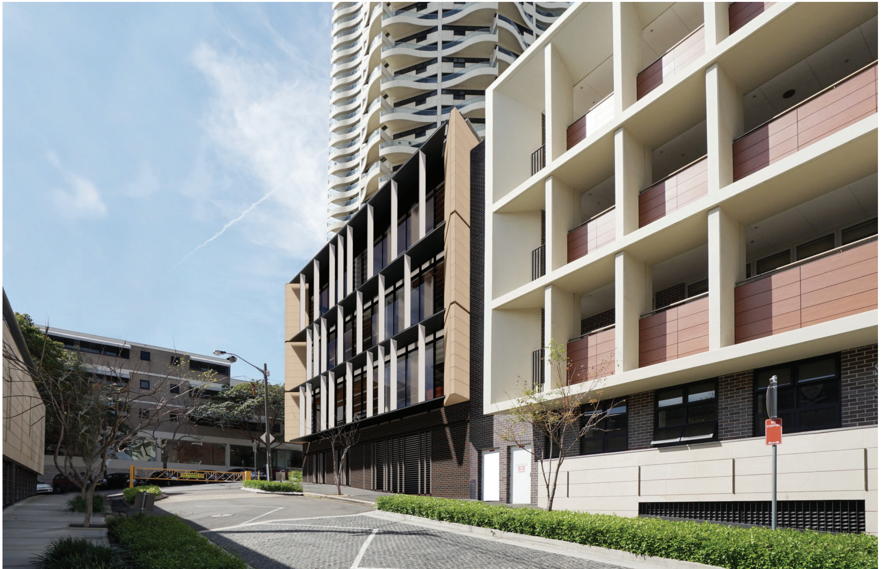
View looking east along St Peters Street
