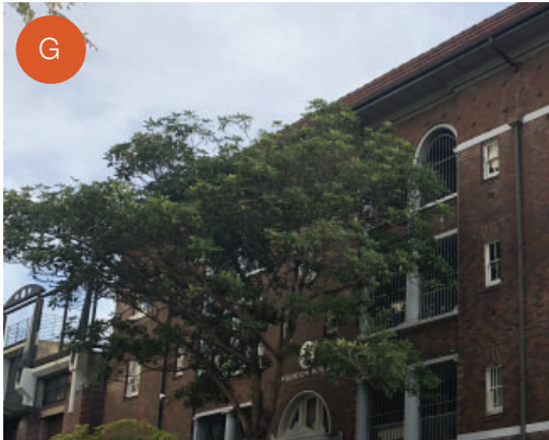
Forbes Street: view west to Wilkinson House corner on St Peters Street intersection
