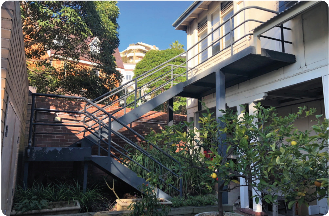
Utilitarian service stair
