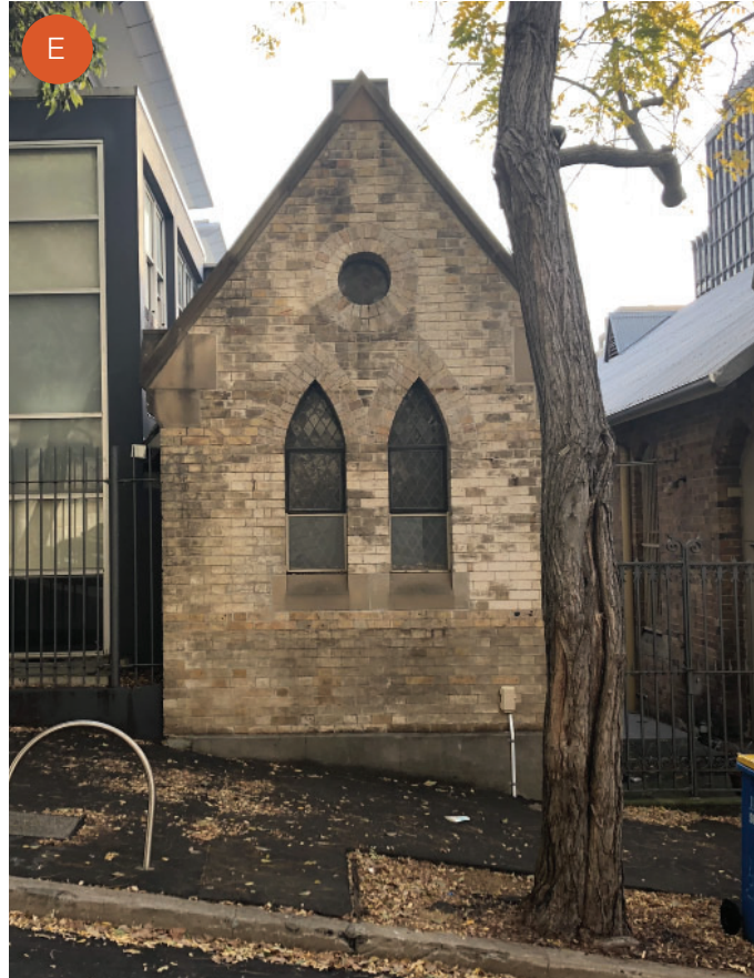
Forbes Street: view west to Diana Bowman Performing Arts Centre and St Peters Parish Hall
