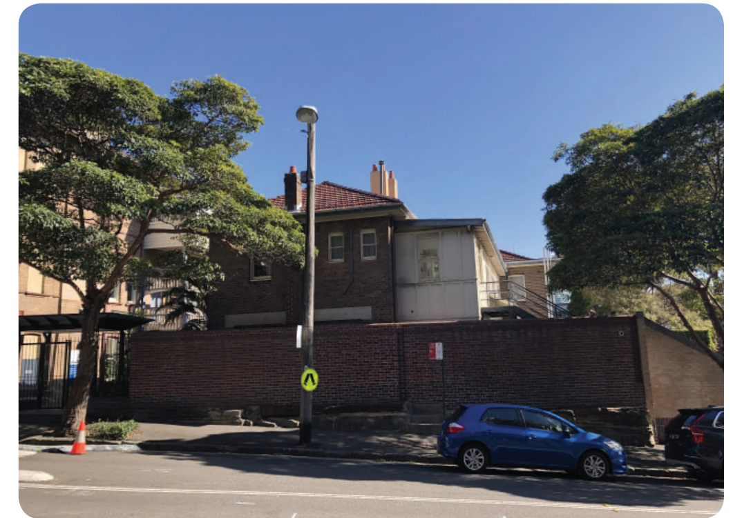
Utilitarian ad hoc additions add little to the streetscape and create a poor sense of entry
