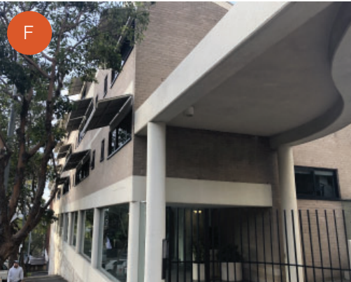
Forbes Street: view east into the Horizon Building complex
