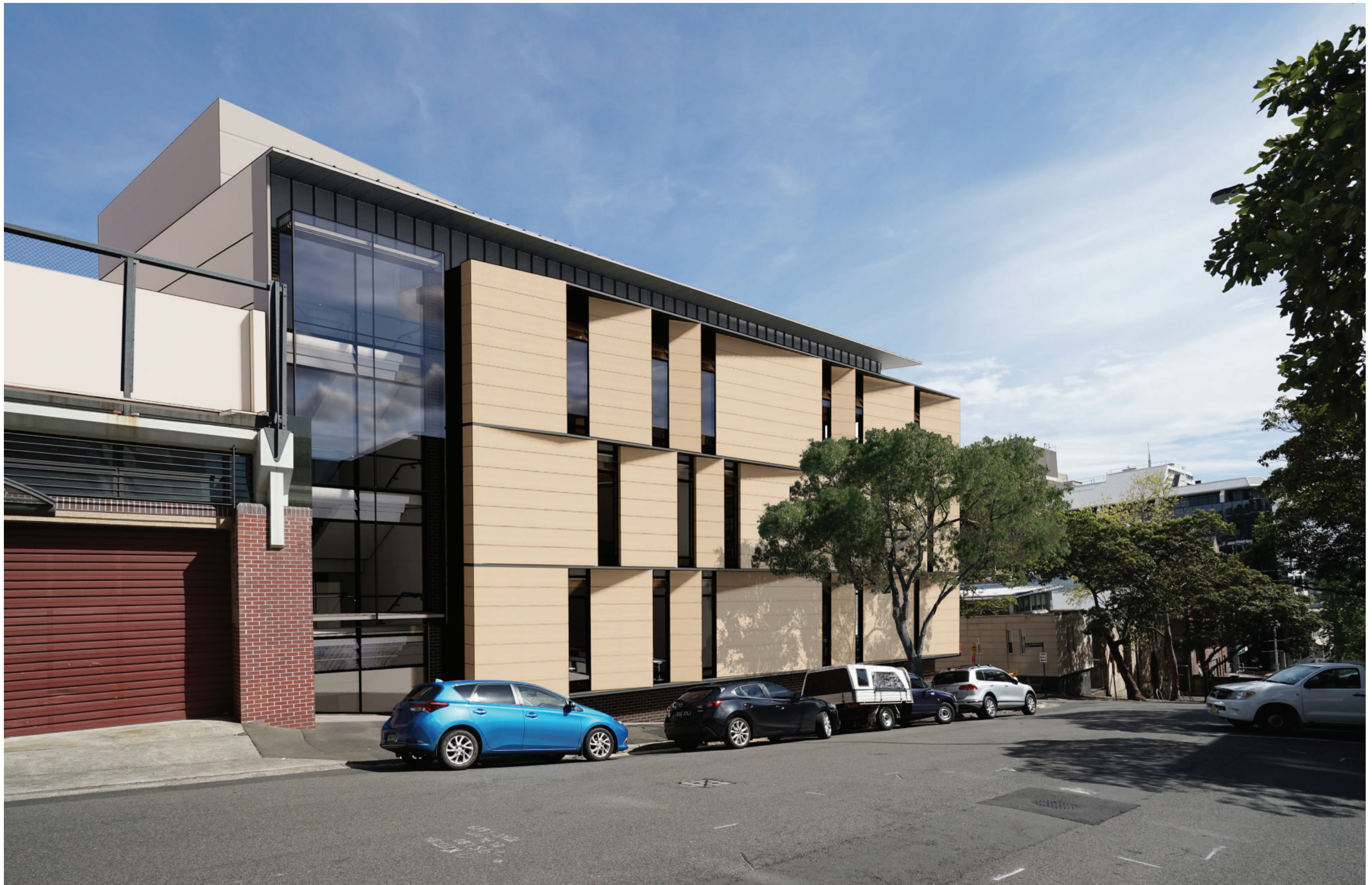
View looking North along Forbes Street
