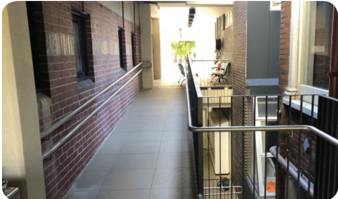
Misaligned floor levels to access Wilkinson House result in convoluted access and a series of narrow ramps.
