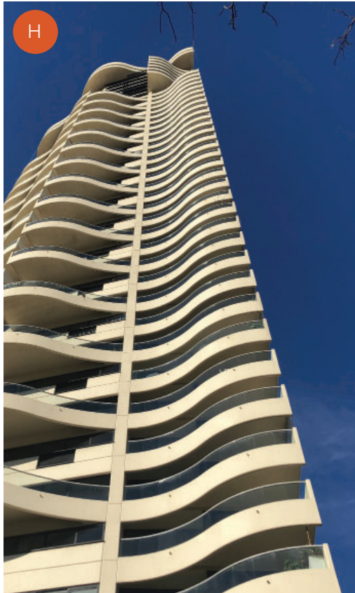
Forbes Street: view east to the Horizon Building tower
