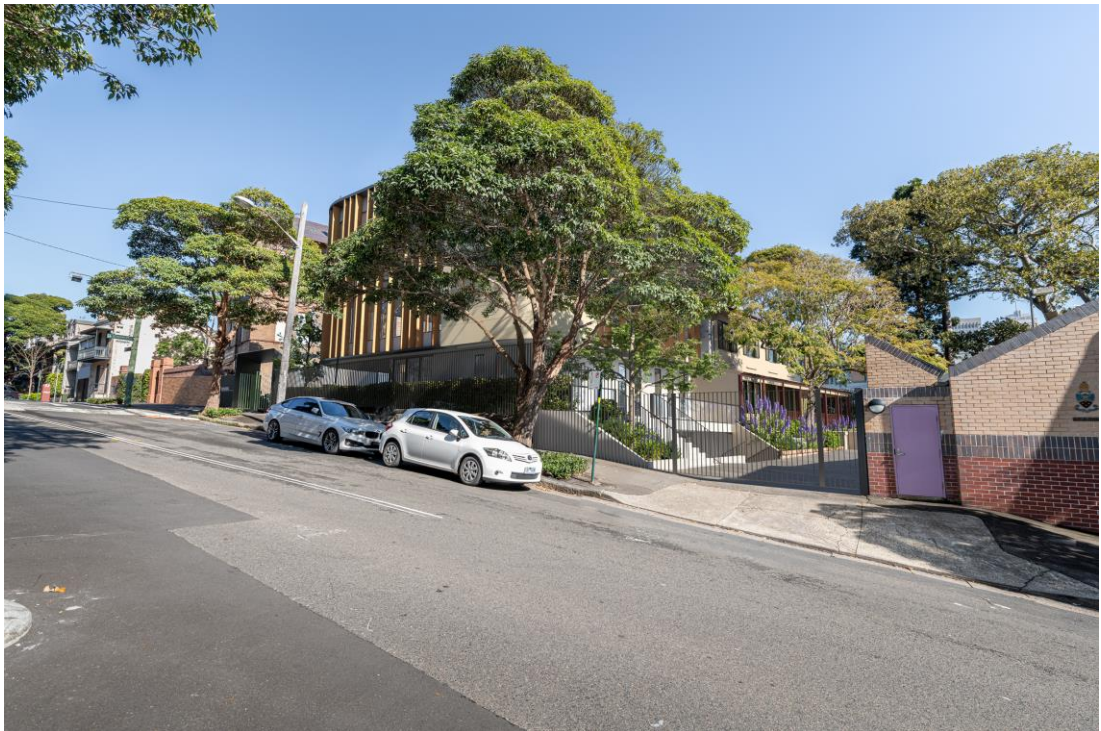
6 View towards the northern elevation of Barham from Forbes Street.
