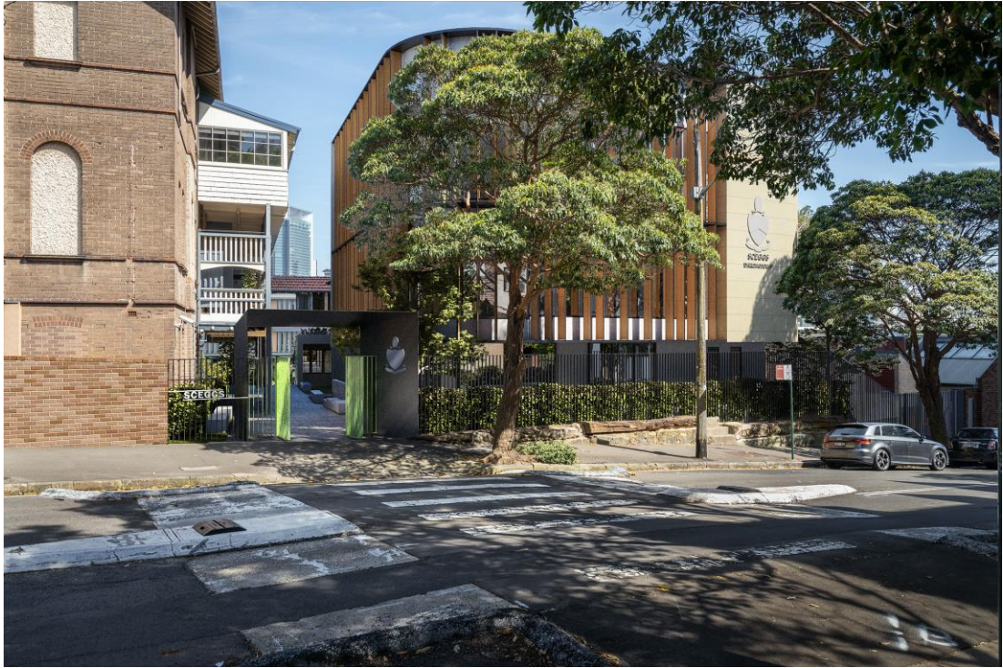
5 View from Forbes Street towards the revised Chapel Building and the south-eastern corner of Barham.
