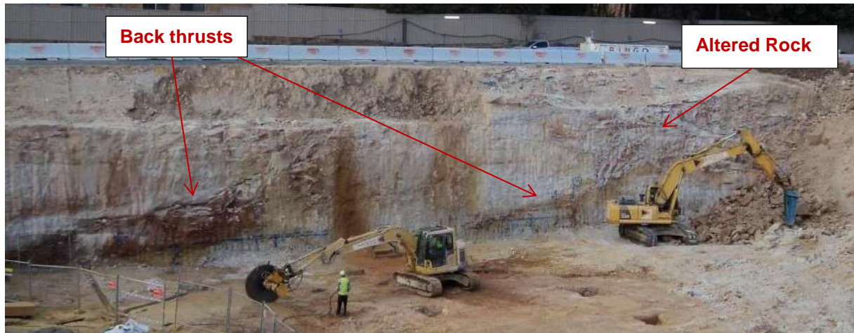
Figure 7: Back thrusts in an excavation wall at a nearby site
