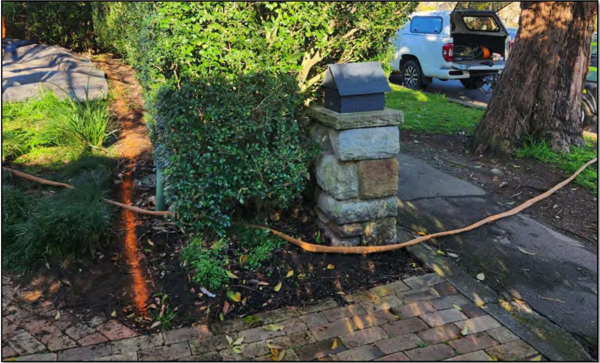
Figure 13 – Location of exploratory root mapping investigation trench within NRZ of Tree 85
