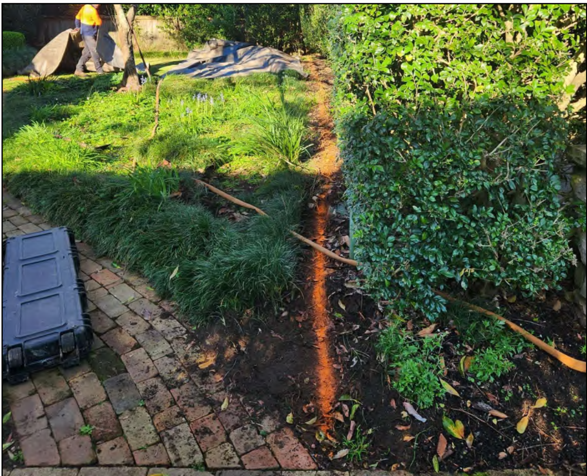
Figure 17 – Location of exploratory root mapping investigation trench within NRZ of Tree 86
