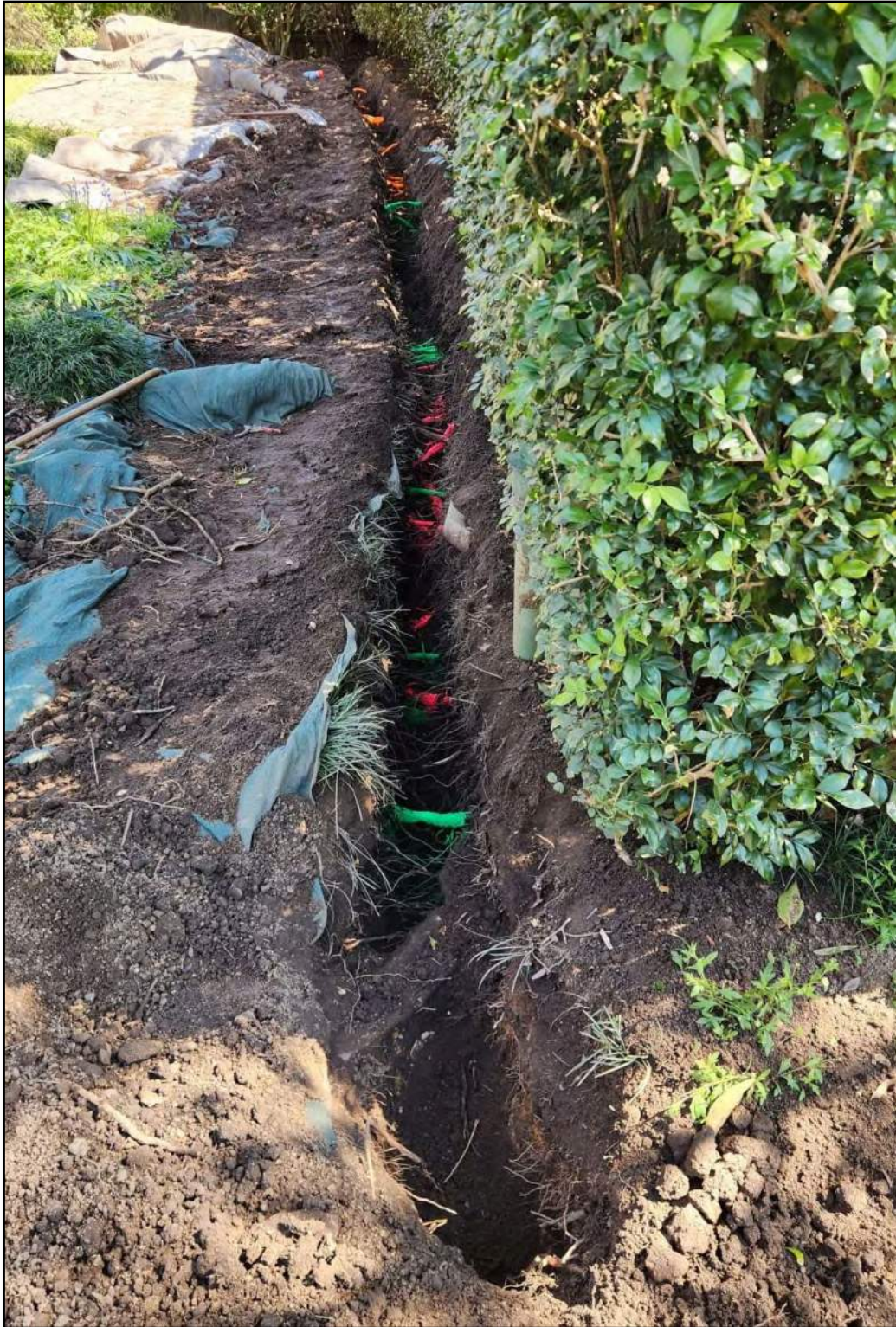
Figure 15 – Roots 4-12 (marked green) within NRZ of Tree 85. Orange roots associated with Tree 86. Pink roots associated with Tree 102.
