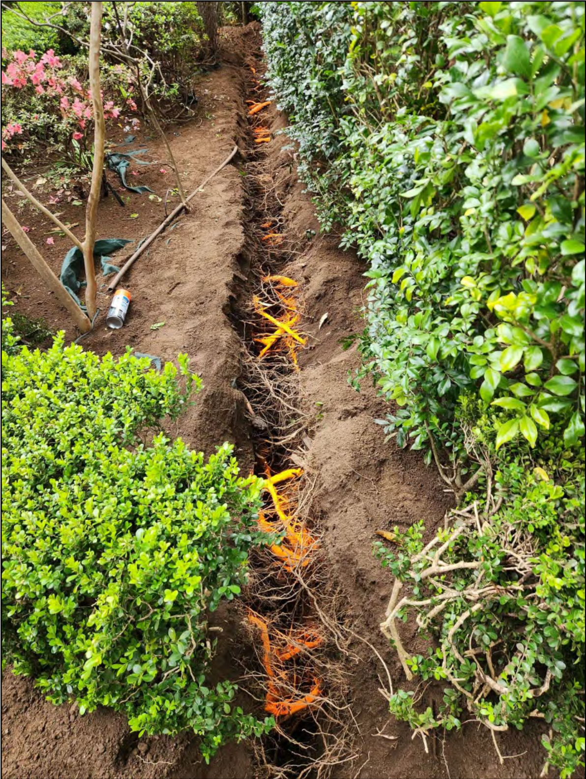
Figure 7 – Location of No. 20 Lord Street front setback root investigation trench within NRZ of Tree 20 showing Roots 1-31
