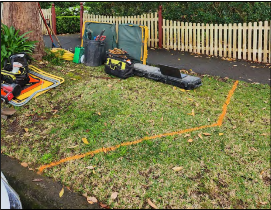
Figure 5 – Location of Lord Street verge root mapping investigation trench within NRZ of Tree 20
