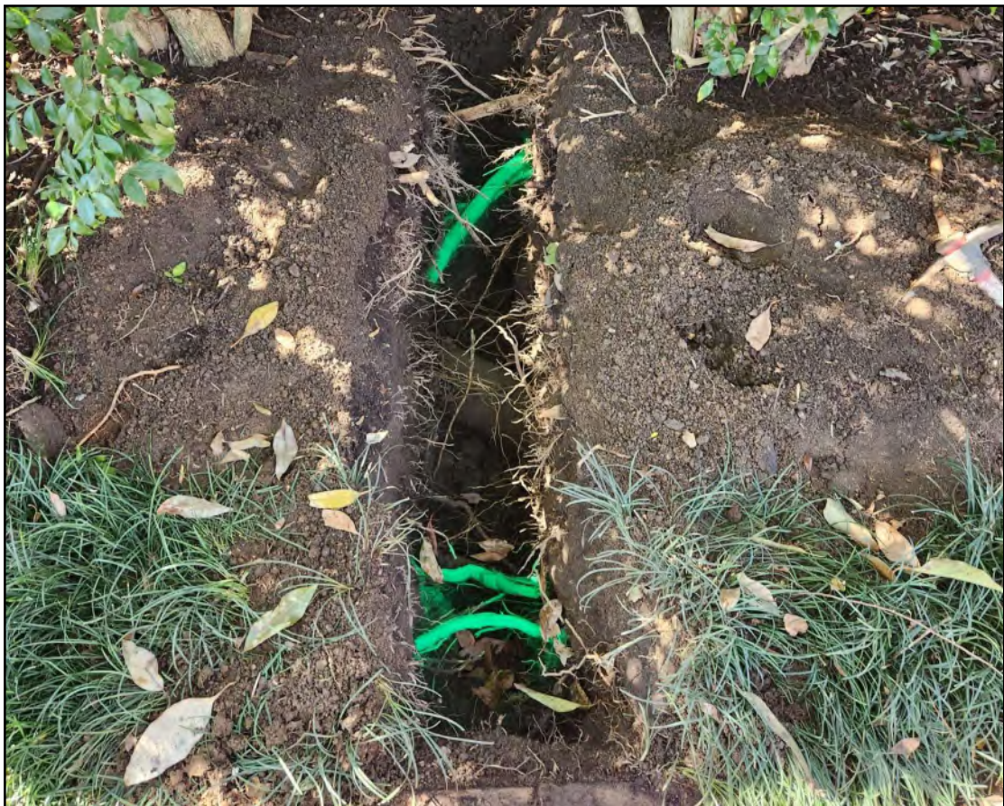
Figure 14 – Roots 1-3 (marked green) within NRZ of Tree 85
