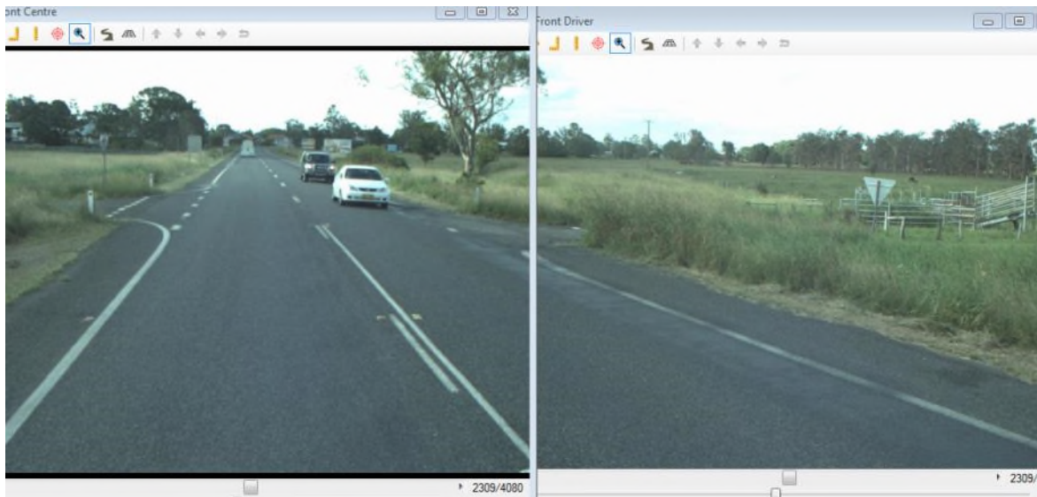
Pacific Highway / Watson Street intersection before upgrade
