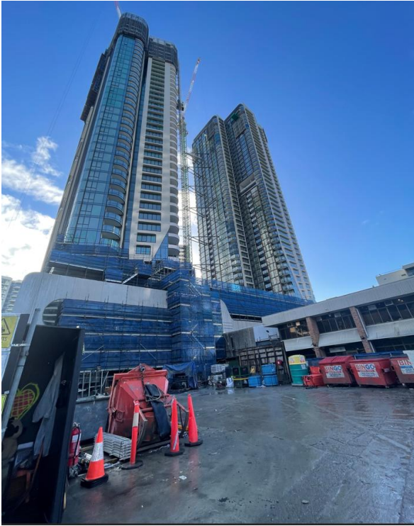
Picture 1 The site as viewed from Marquet Street
