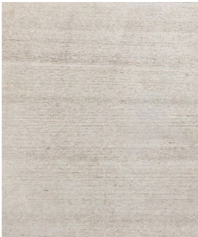
Concrete Paving Broom Finish
