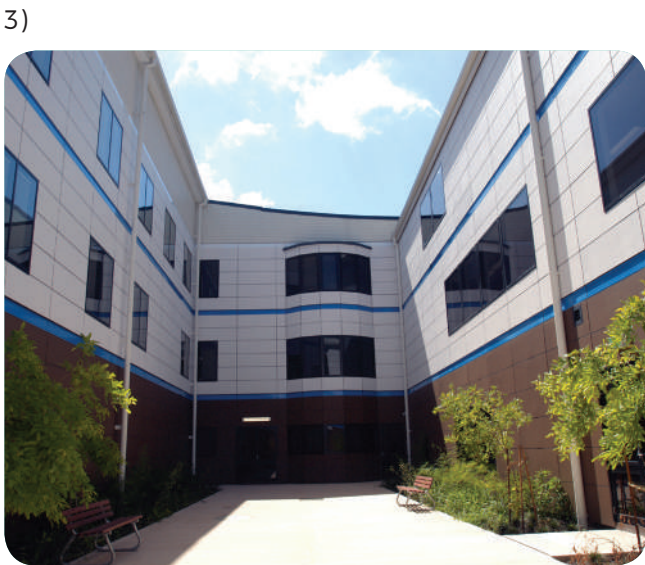
INTERNAL COURTYARD OF BLOCK A
