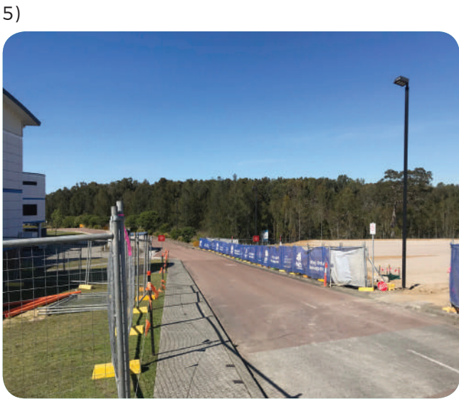
VIEW SHOWING THE RING ROAD WHERE THE OVER BRIDGE WILL CONNECT TO THE EXISTING HOSPITAL ON THE LEFT
