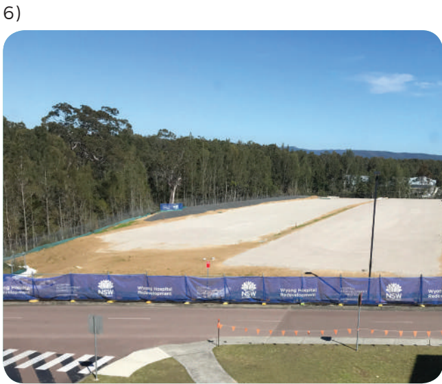
VIEW FROM LEVEL 3 CORRIDOR OF BLOCK A LOOKING OVER THE HOSPITAL EXTENSION SITE SHOWING THE DENSE EXISTING VEGETATION AND THE YENGO NATIONAL PARK IN THE DISTANCE
