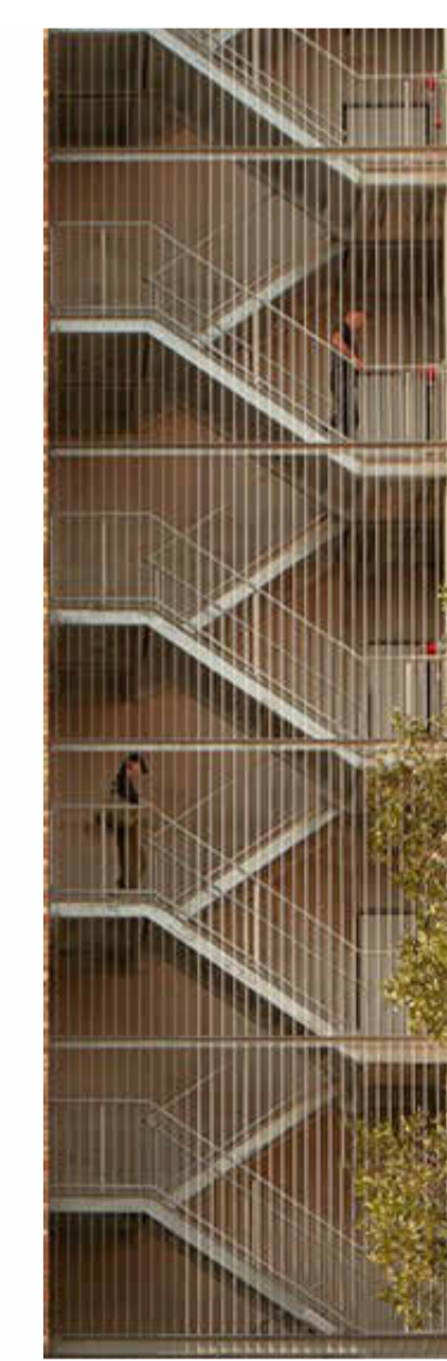
08 Louvred Screening Green / Red Tone BUILDING A AND B
