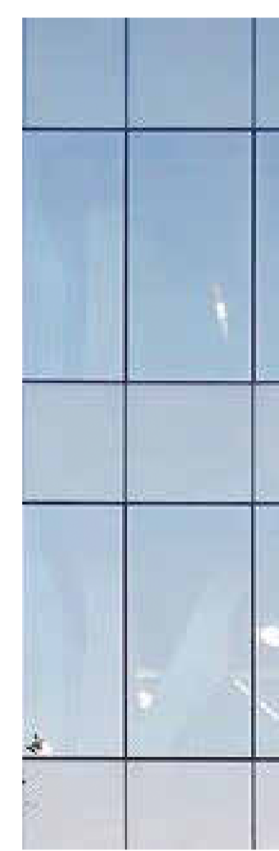
07 Window Wall Clear Glazing BUILDING A AND B
