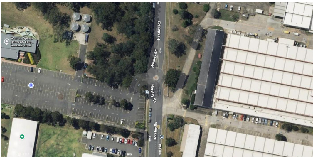
Figure 7 Aerial image of the existing Horsley Road Intersection
