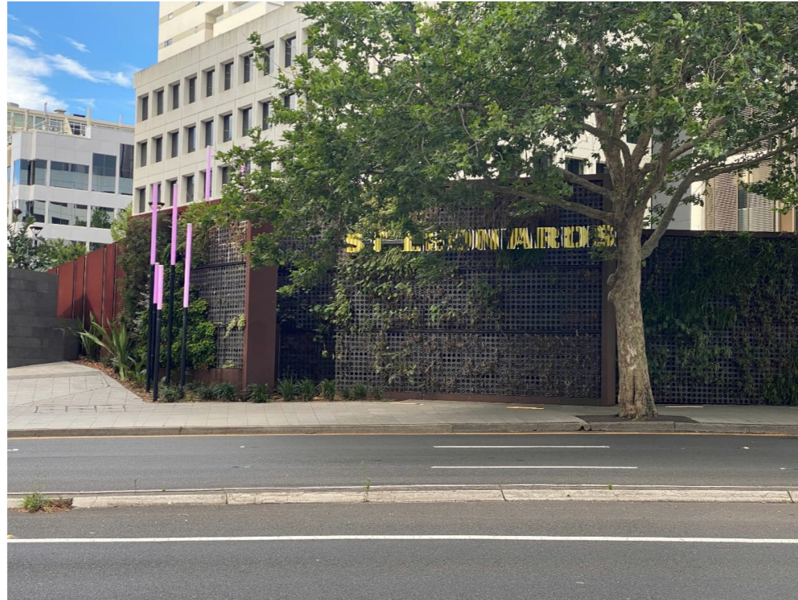
Mitchell Street Square – failed greenwall with westerly aspect
