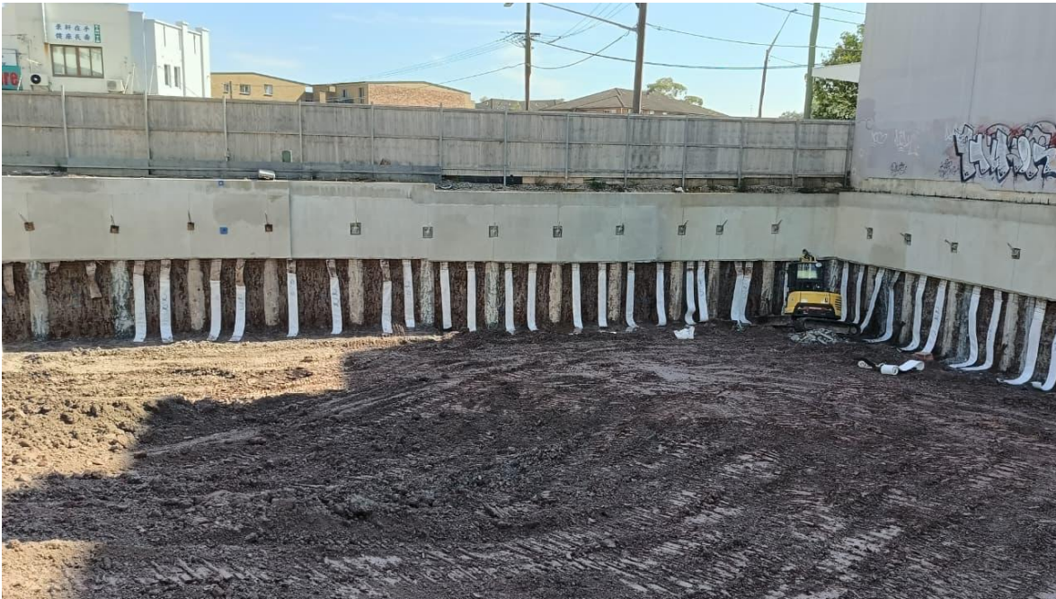
Figure 18. Shoring wall construction for Basement, Southern part of the site.
