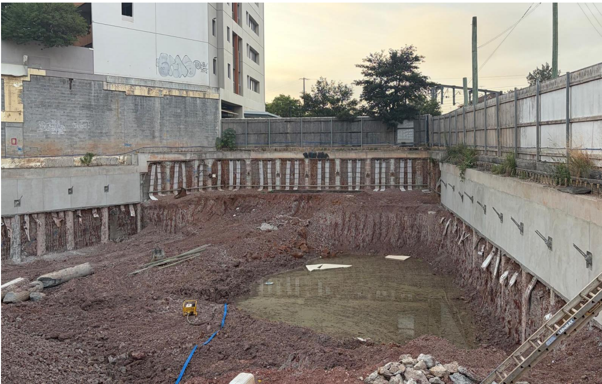
Figure 19. Shoring Wall construction, Northern part of the site.
