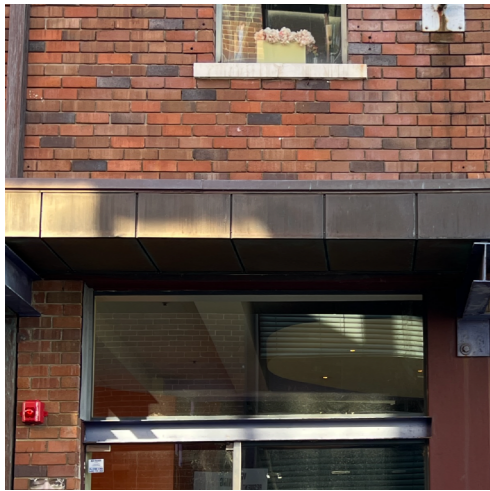
RSC - Copper awning
