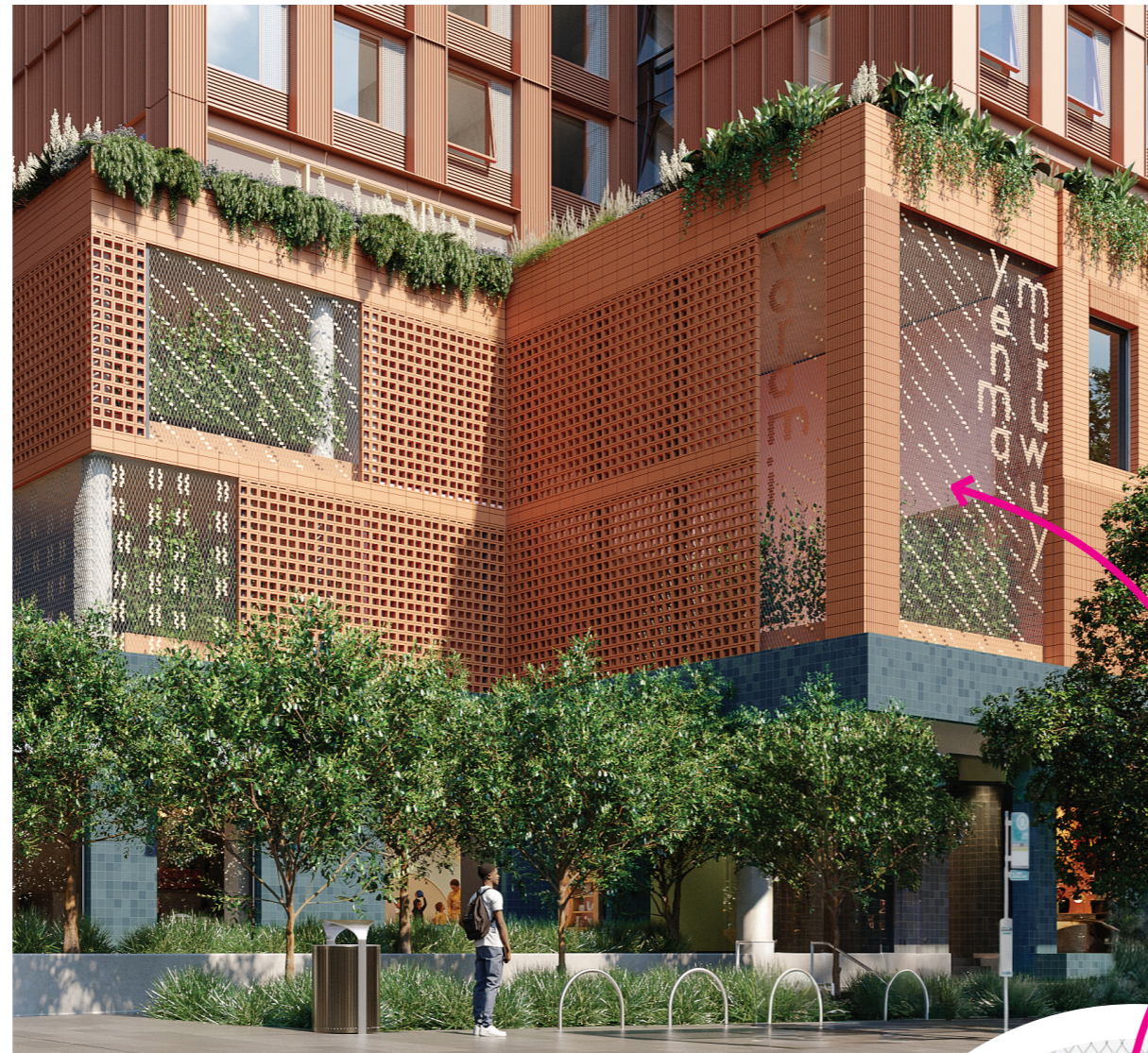
View 1 - Street view of mesh screens at outdoor play space openings
