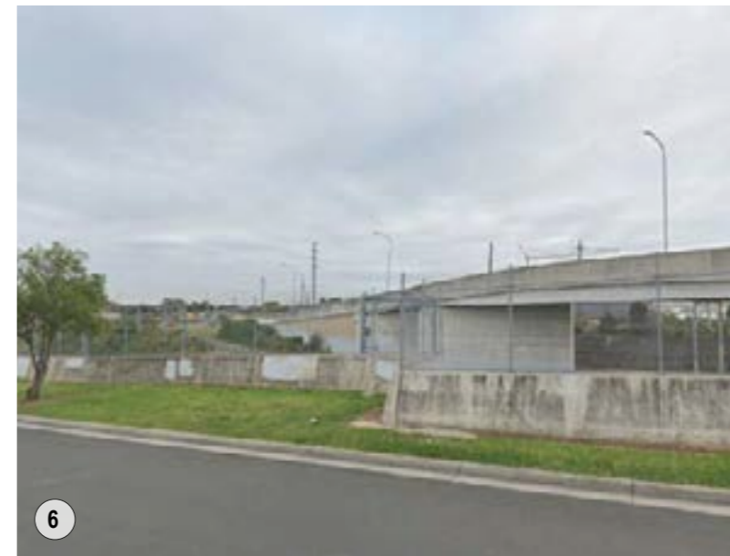
6 VIEW OF SITE FROM WELLINGTON ROAD - RAILWAY SERVICE BRIDGE IN FOREGROUND
