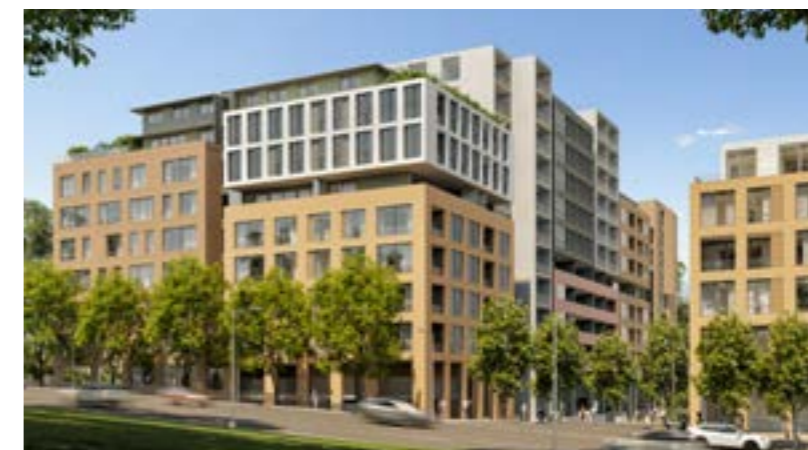
VIEW FROM AUBURN ROAD
