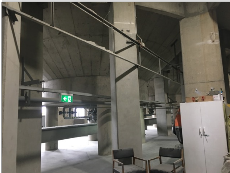
Figure 13: The conical base of the silos visible underneath.
