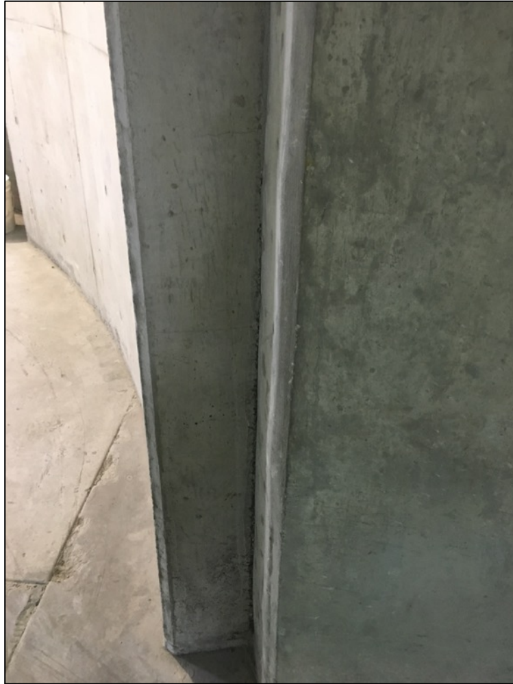
Figure 25: The 300mm thick reinforced concrete ring.
