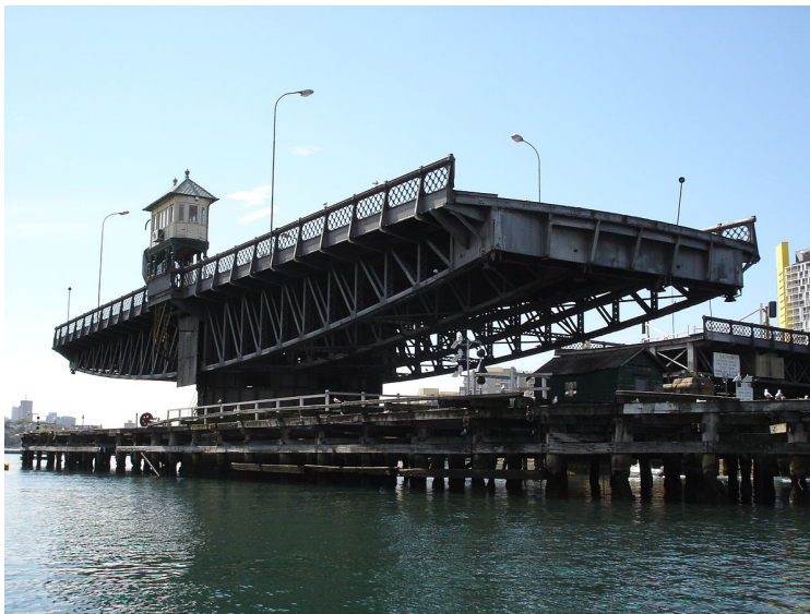
Figure 18: The Glebe Island Bridge, to the east of the site.
