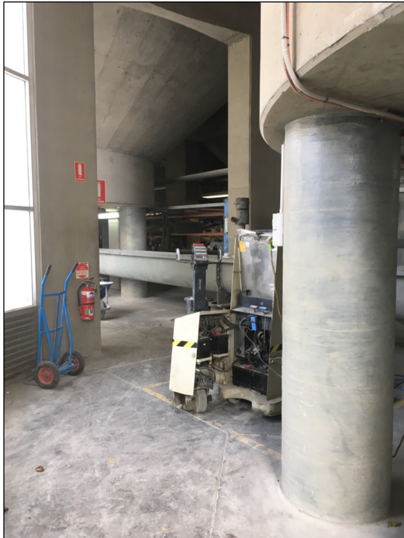
Figure 15: The conical base of the silos visible underneath.
