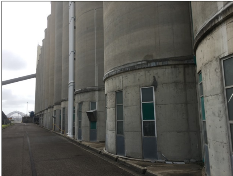
Figure 11: The unpainted northern elevation of the silos.
