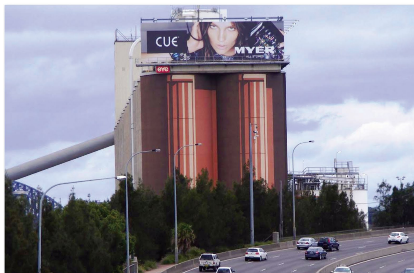
Figure 28: View of the silos in Anzac Bridge.
