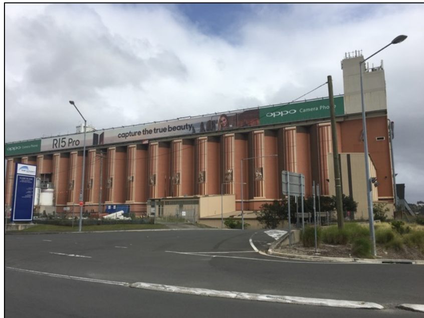
Figure 30: View of the Glebe Island Silos from southern side of Sommerville Road.
