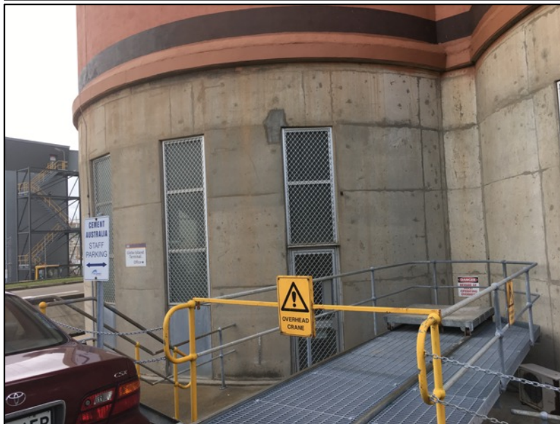
Figure 12: Access to the site offices on the western elevation.
