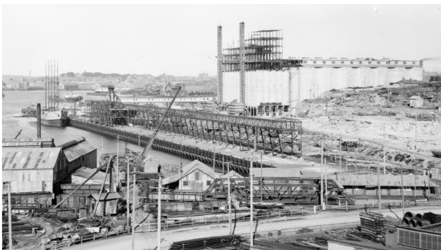
Figure 5: The Glebe Island Silos in the 1920s when they were used for storing wheat.
