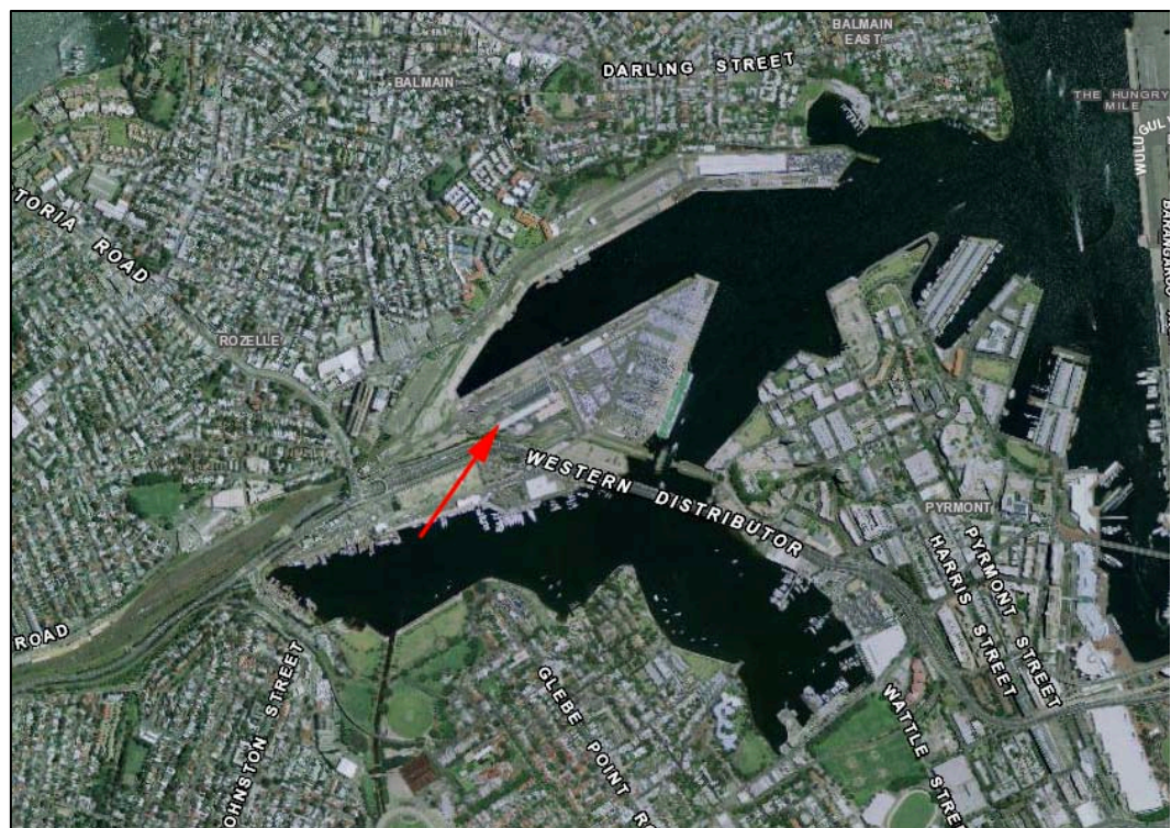
Figure 16: Aerial photograph over the site and the surrounding area.
