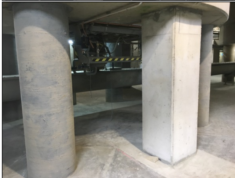
Figure 24: New square footings at the base of the silos.
