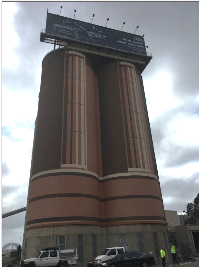
Figure 10: The western elevation of the silos.
