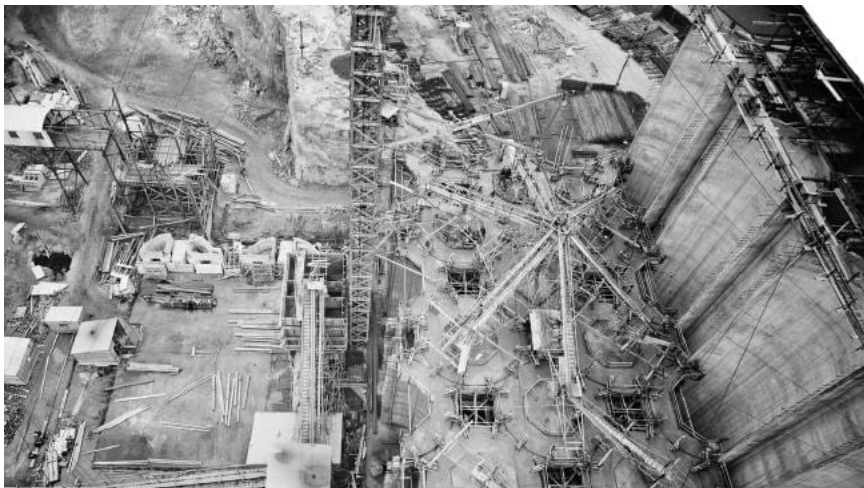
Figure 4: The Silos under construction in the 1920s.
