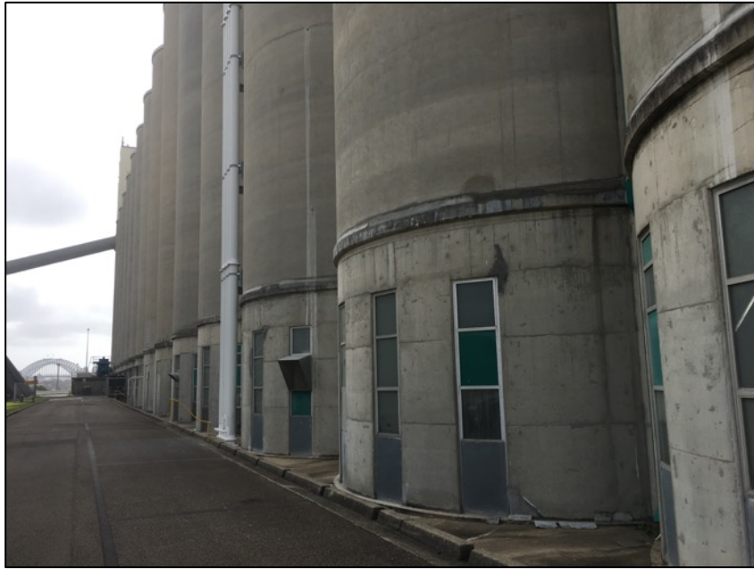
Figure 31: The northern side of the Glebe Island Silos viewed from Sommerville Road. Note the Sydney Harbour Bridge in the distance.
