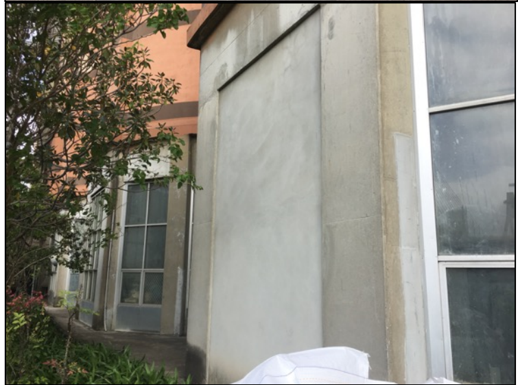
Figure 22: Infilled window bay on the southern side of the silos
