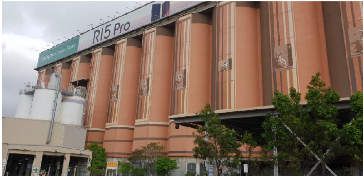
Figure 2- Glebe Island Silos, looking north-west
