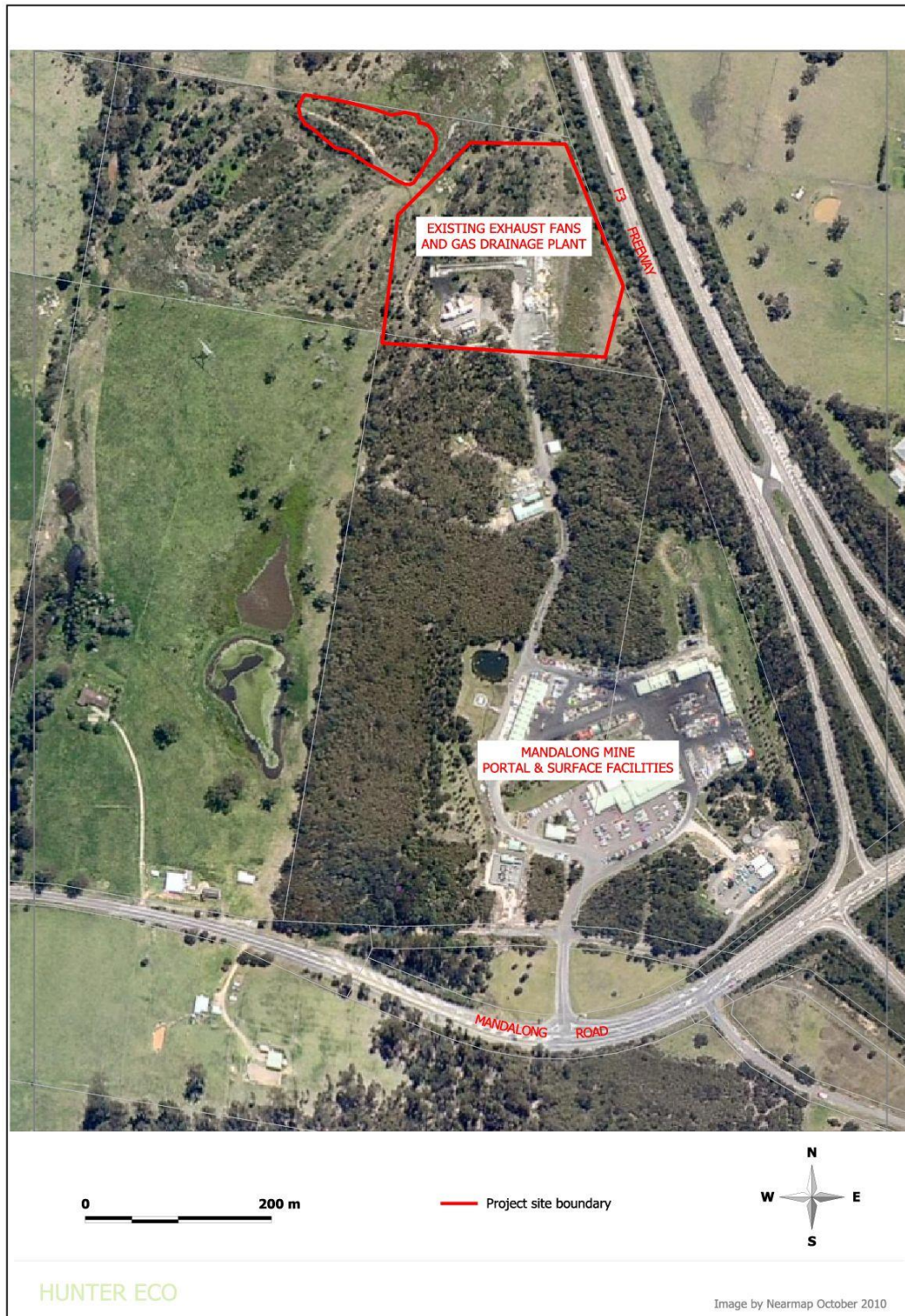
Figure 1 The Mandalong mine surface facilities and proposed project site
