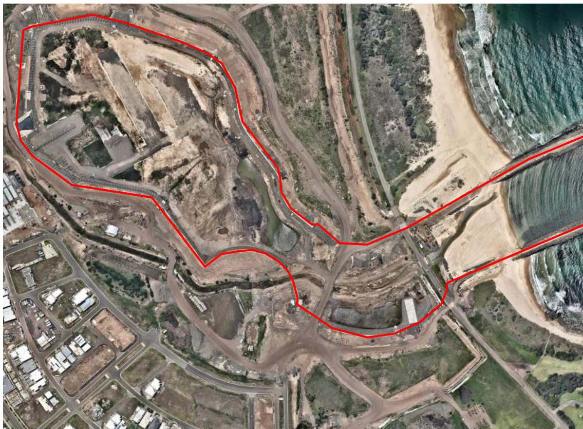
Figure 1 – Aerial Image of Shell Cove Boat Harbour & Marina
