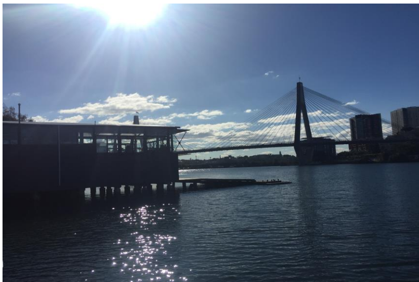
Figure 6 - Adjoining the site to the east is the Blackwattle Bay Marina
