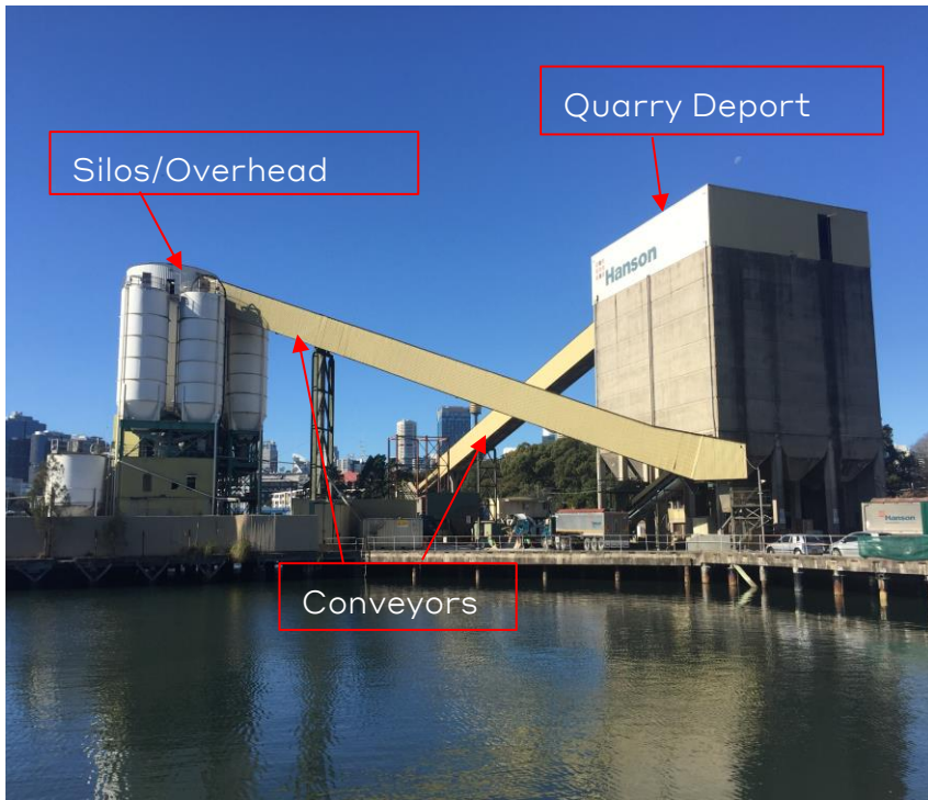
Figure 5 - View of the existing concrete batching plant, looking east from the foreshore public footpath
