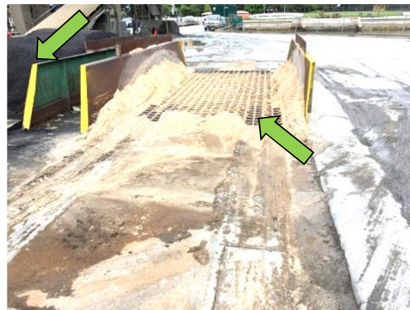
Photo 12: Ground bin for collection and storage of delivered concrete raw materials such as sand and aggregate.
