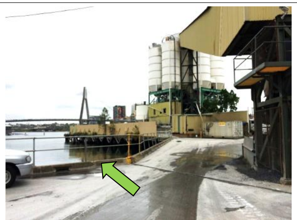
Photo 5: Raised edges/curbing surrounding the site prevents direct stormwater flow into Blackwattle Bay
