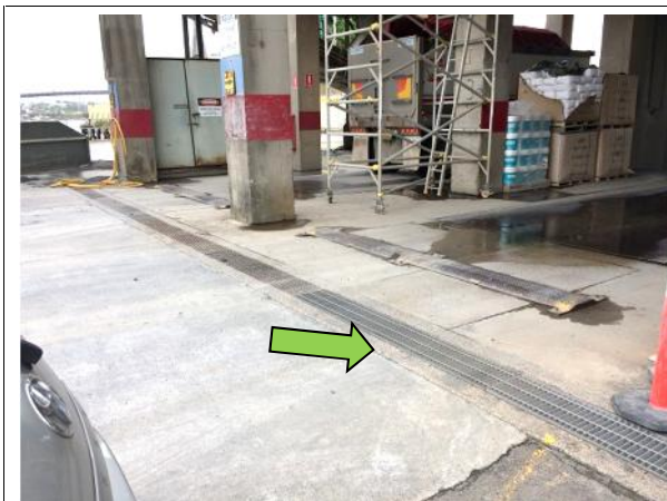
Photo 4: Stormwater drainage at the exit to the Quarry Depot/Weighbridge area
