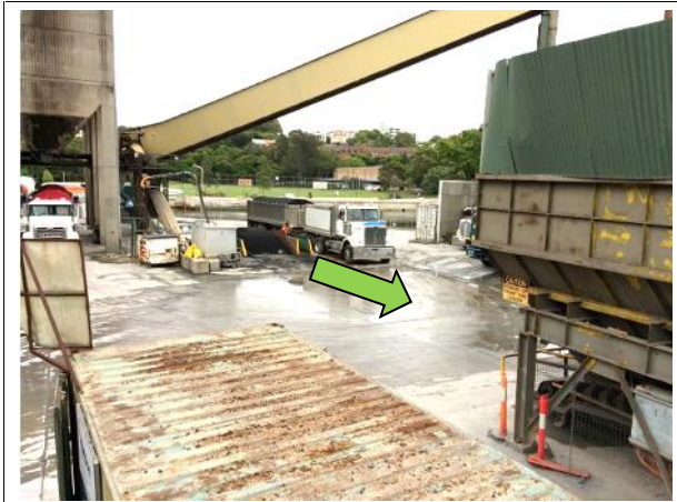
Photo 3: Graded area used to wash down the exterior of the trucks
