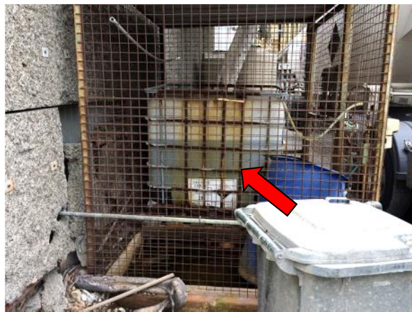
Photo 18: Acid stored next to the truck access to the processing area
