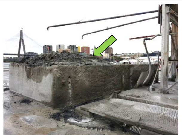
Photo 9: Solid slurry stored in bins next to the washout pits
