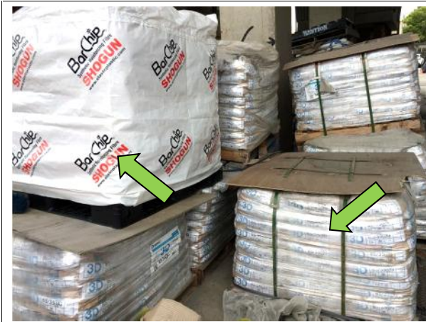
Photo 16: Concrete additives stored on site
